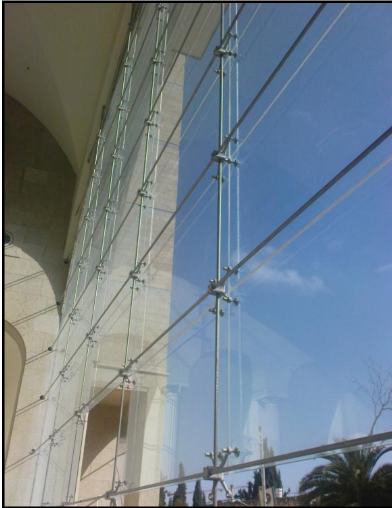
Figure 2.21. The Example of Aluminium Glass Curtain Wall System (Source: Alumil Curtain Wall Catalog, 2011)
