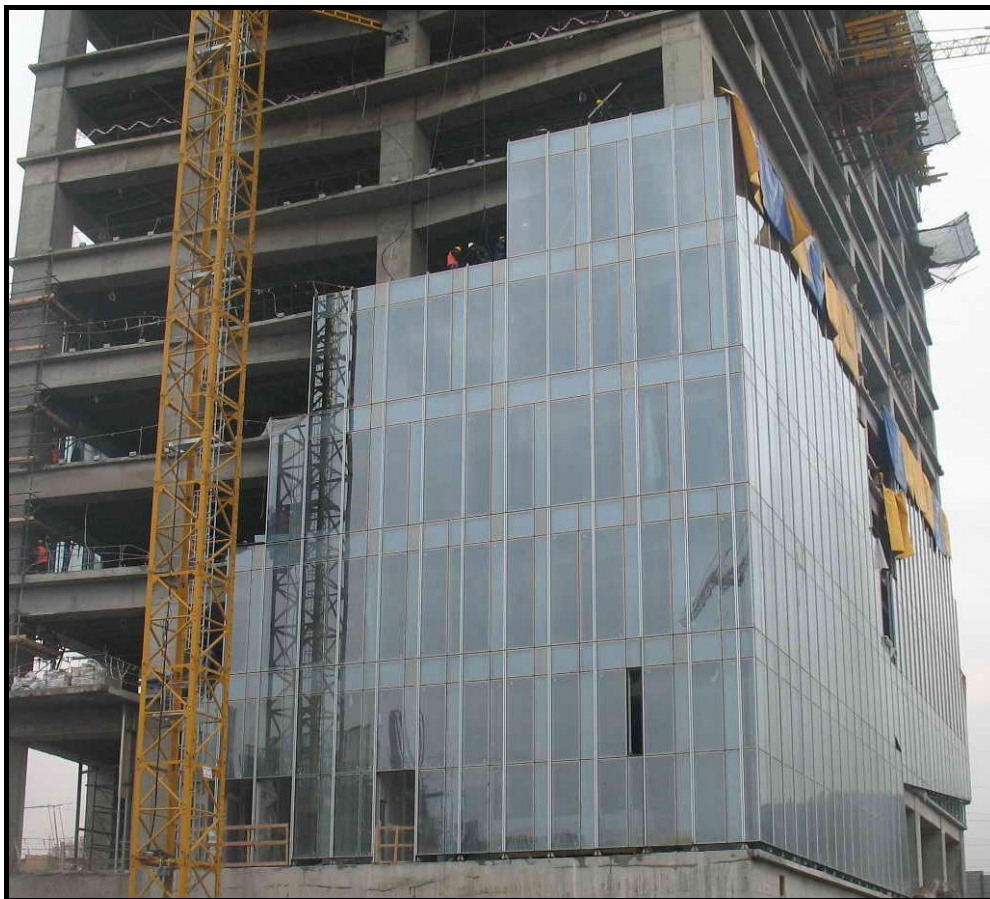
Figure 2.28. The Installation of Units From Bottom to The Top, Esentai Tower (Source: Feniş System, 2012)
