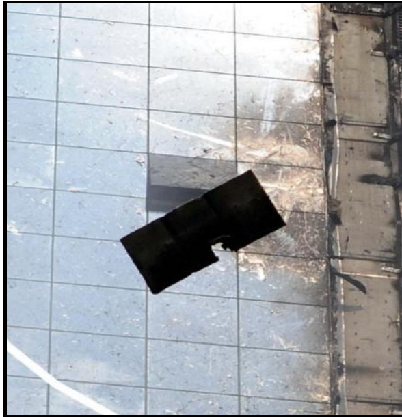
Figure 2.38. The View From The Fire In Polat Tower, Şişli, İstanbul. (Source:www.hurriyet.com.tr,16.07.2012)
