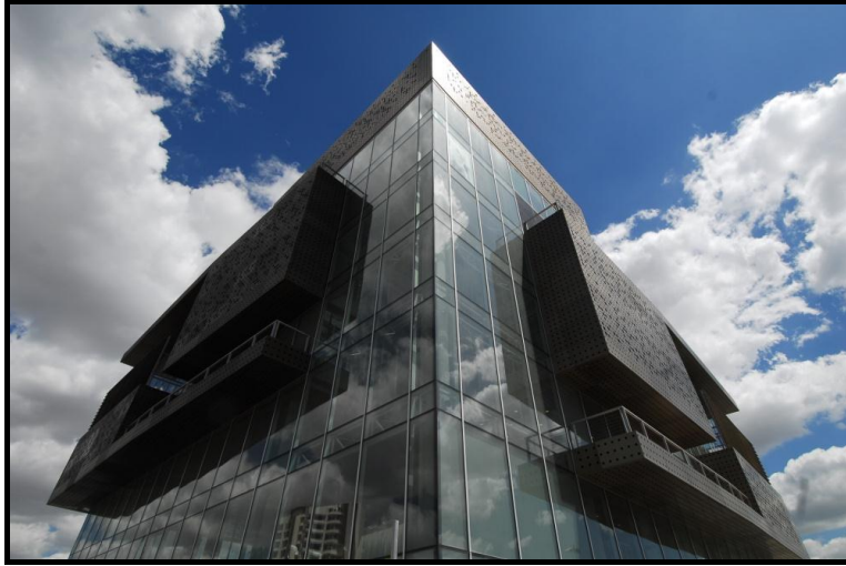
Figure 2.15. Doğan Medya Center, Ankara (Two-sided Conventional Aluminium Curtain Wall System) (Source:Alumil, 2011)
