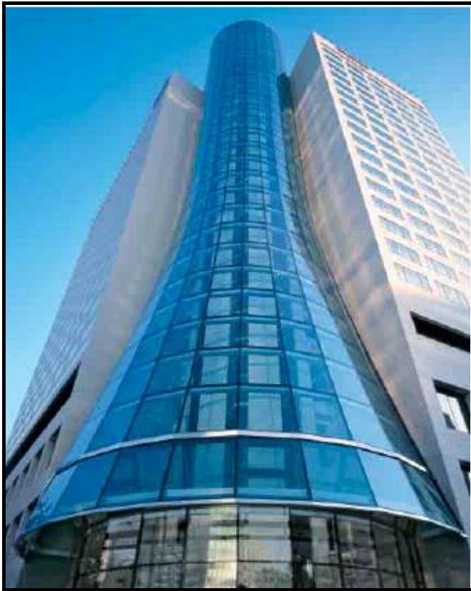
Figure 2.19. Structural Glazing Curtain Wall Sytem, Westin Hotel, Poland (Source: Shücco Curtain Wall Catalog, 2011)
