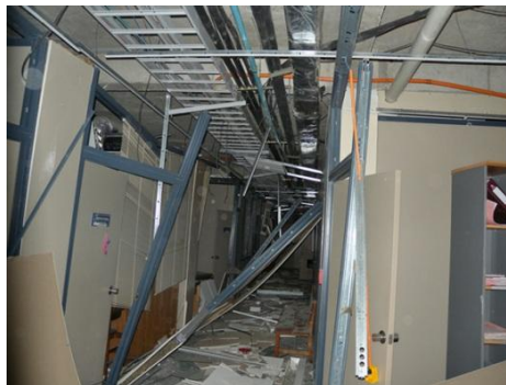
Figure 3.16 The damage caused by the collapse of the suspended ceiling
