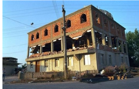
Figure 3.18 A building infill walls of which collapsed after the 1999 Marmara Earthquake
