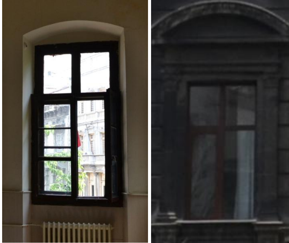
Figure 15: a) Interior view of a window opening, Zapyon R.İ.O.L. It is seen that the opening is spanned with a segmental arch. b) Exterior view of the window opening, Zapyon R.İ.O.L. From outside the opening is perceived to be spanned with a lintel (Author, June 2011).
