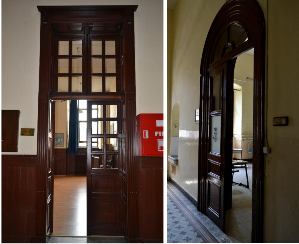
Figure 16: a) Door opening of a classroom in Zoğrafyon R.L.İ.O., which is spanned with lintel. b) Door opening of a classroom in Zapyon R.İ.O.L., which is spanned with a central arch. (Author, June 2011).
