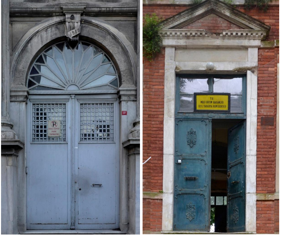
Figure 17: a) Entrance door of Maraşlı R.İ.O.; spannd with arch, different than interior doors which are spanned with lintel. b) Entrance door of Tarabya R.İ.O.; made of metal, different than timbr framed inteiror doors.
