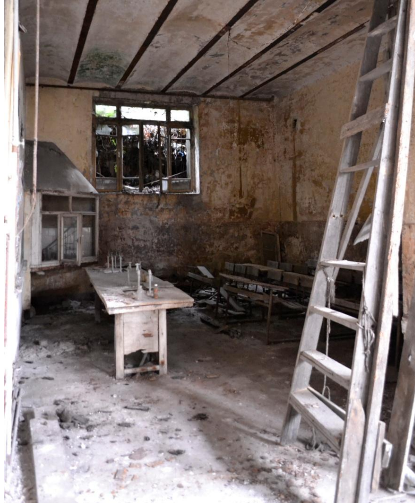
Figure 21: View of a laboratory space, Merkez R.İ.O.L. The broken window frames causes more deterioration inside.
