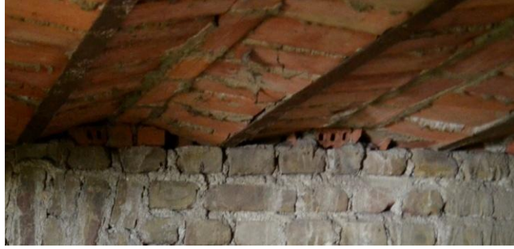
Figure 19: Detail view of brick arch floor, Tarabya R.İ.O. (Author, June 2011).
