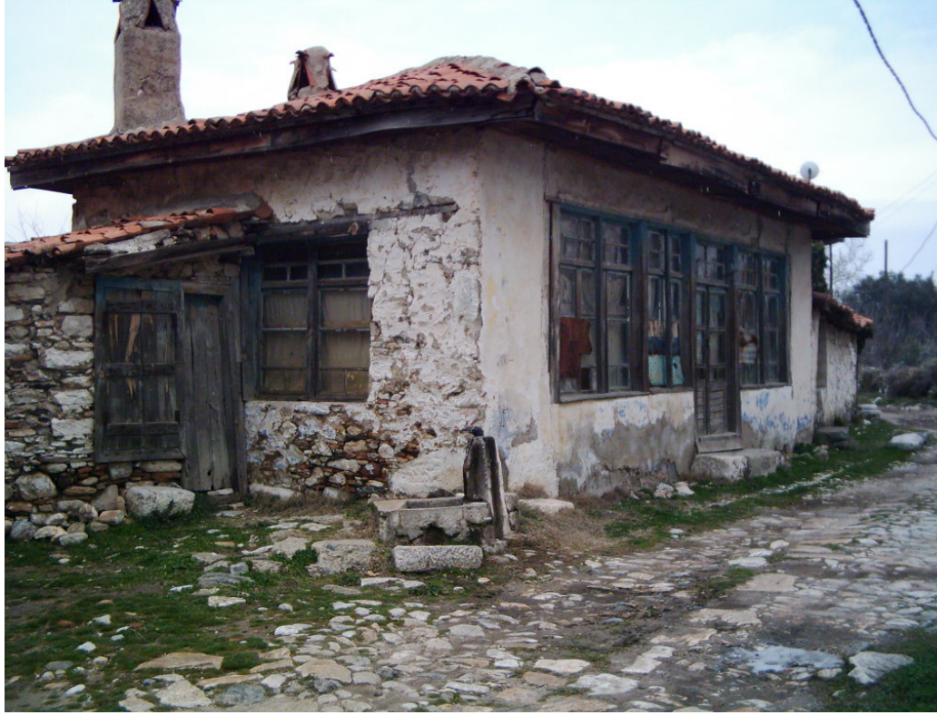
Figure 3.12. Traditional commercial building
