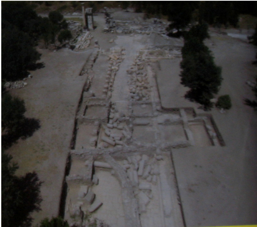
Figure 3.50. Excavation of the colonnade road
