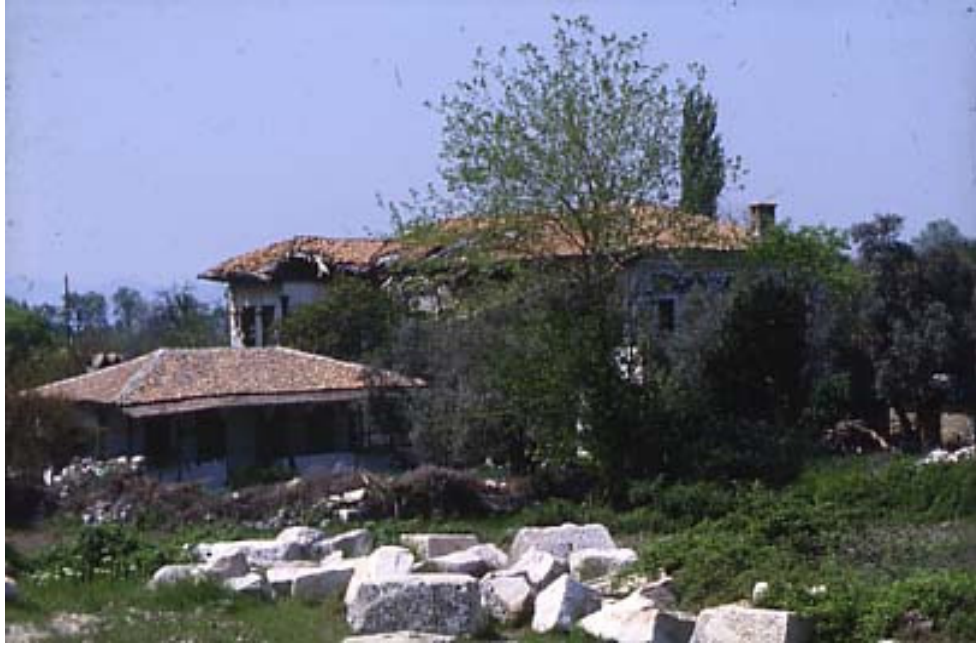
Figure A17- North façade of Abdullah Ağa's mansion in 1993 (Archive of General Directory of Cultural Heritage and Museums)
