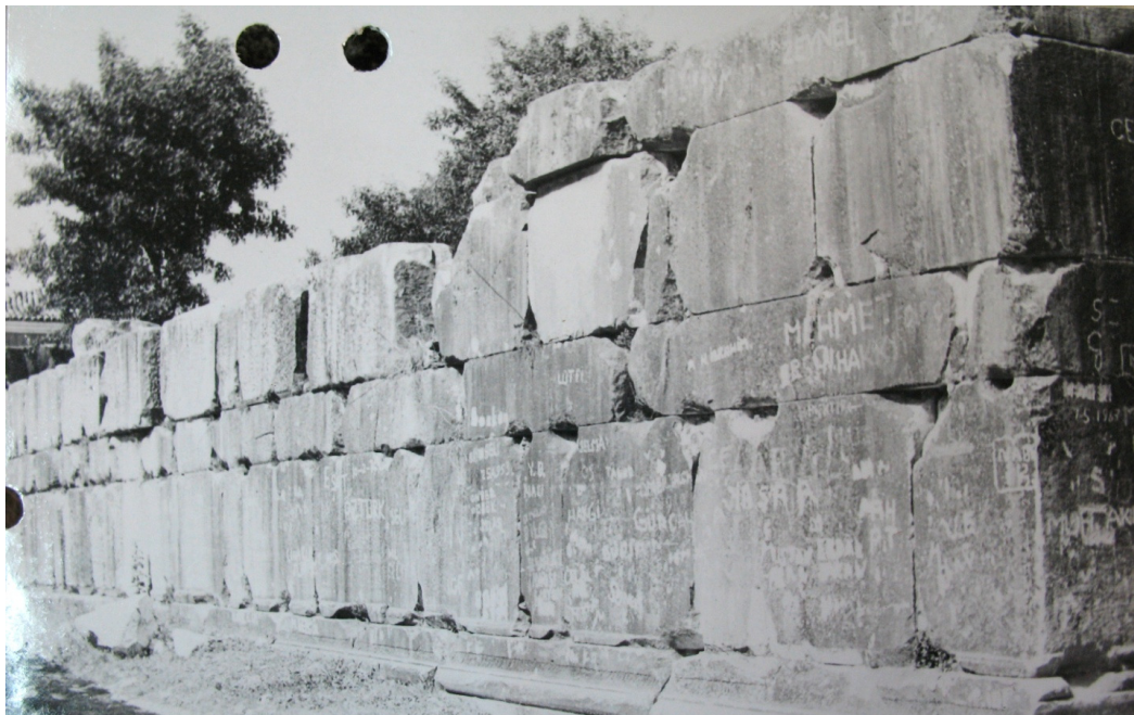
Figure A4- Bouleuterion in 1972 (Archive of General Directory of Cultural Heritage and Museums)
