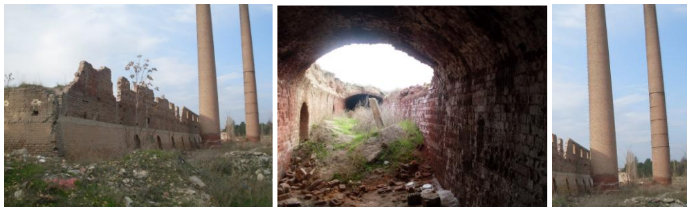
Figure 100: a) Demolishment of the roof and some parts of the exterior walls in the Kiln Building 1 (author, March 2010) b) Destruction on the upper parts of the vaults and walls in the Kiln Building 2 (author, March 2010) c) Dampness rising from the ground on the smokestack (author, March 2010)
