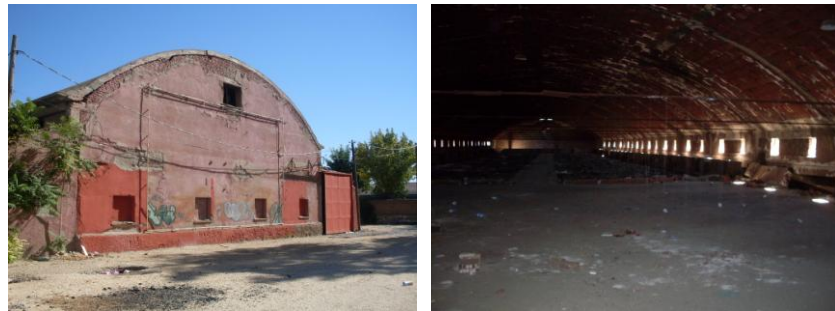
Figure 89: The vault system of the factory (author, March 2010)
