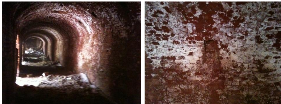
Figure 99: The dampness problem in the interior of the Kiln Building 2 (author, November 2011)
