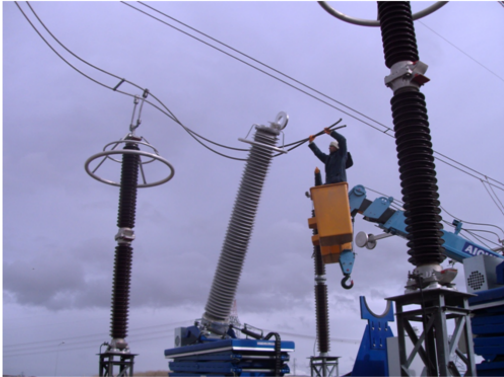
Figure 1.2: Cutting of high voltage lines
