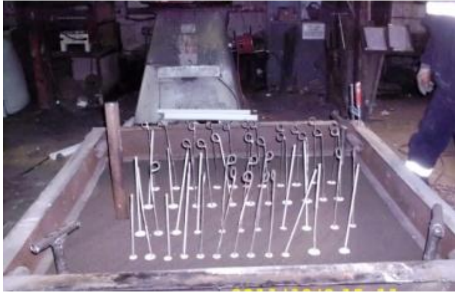
Figure 4.5 Formation of the Gas Release Holes
