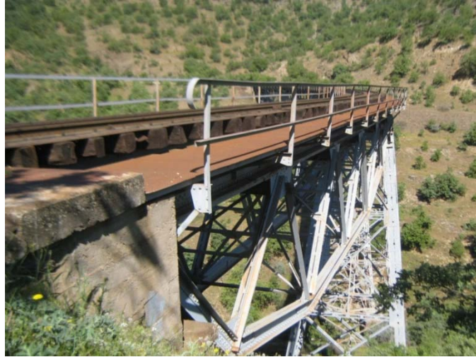
Figure 2.6: Bridge horizontal curve, vertical slope and super elevation view
