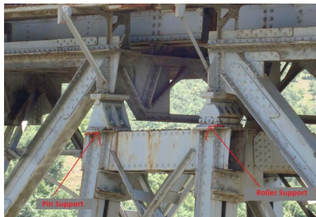
Figure 2.7: Bridge trusses supports
