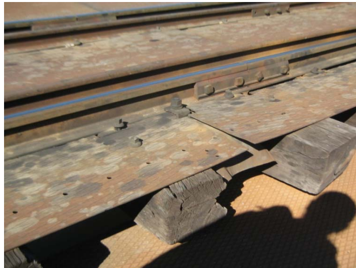
Figure 2.5: Railroad wood sleepers and protective sheet metals
