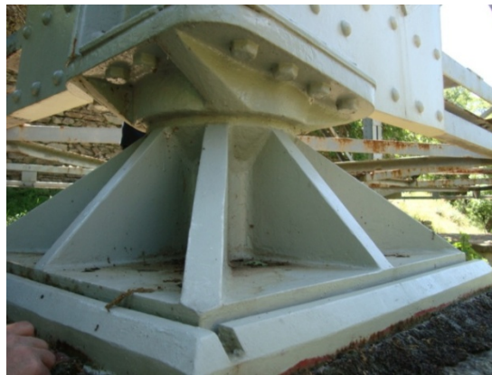
Figure 2.11: Transverse direction moving roller support
