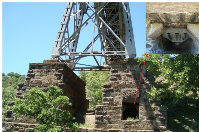
Figure 2.12: Foundation anchorage
