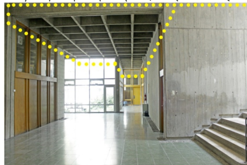
diagram of homogeneity | homogeneous space repeating elements | waffle slab ceiling highlighted
