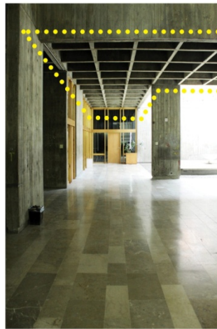
diagram of homogeneity | homogeneous space repeating elements | waffle slab ceiling highlighted
