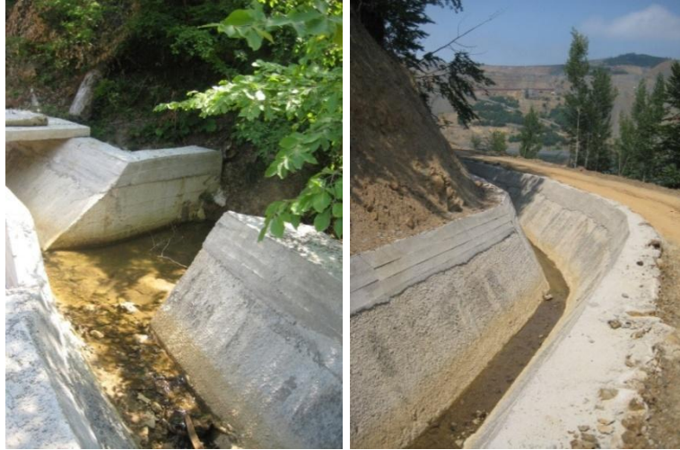
Figure 3.6 Diversion channels behind the dam
