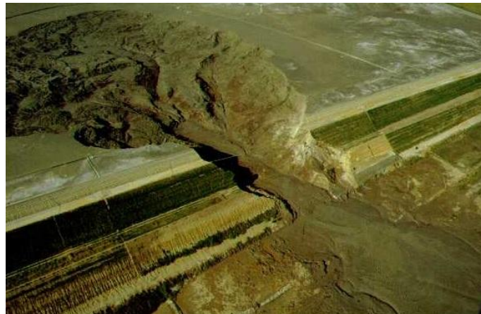
Figure 2.13 Overtopping failure of Merriespruit tailings dam in Virginia, South Africa ( www.tailings.info , 2012)
