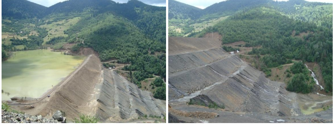
Figure 3.5 Piping through dam because of heavy rain (July 19, 2009)
