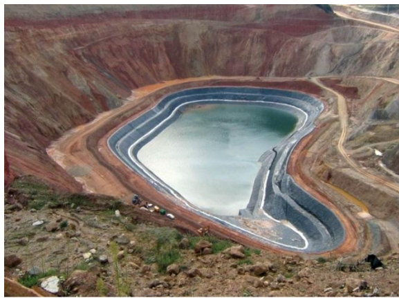
Figure 2.7 The El Valle tailings impoundment (Spain) at startup of tailings disposal operations (In pit type tailings impoundment) (Breitenbach, 2010)
