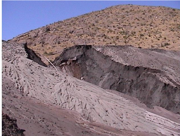
Figure 2.12 Erosion of embankment face of Cerro Negro tailings dam near Santiago, Chile (www.tailings.info, 2012)
