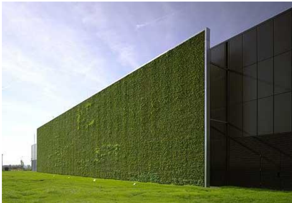
Figure 4.3: A Green Wall Application
