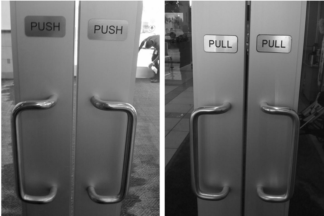
Figure 1.2: Example of the same door handles on both sides of the door where push and pull labels are required ( http://chriselyea.com/design-lessons-learned/badly-designed-doors/ retrieved 18 July 2012)
