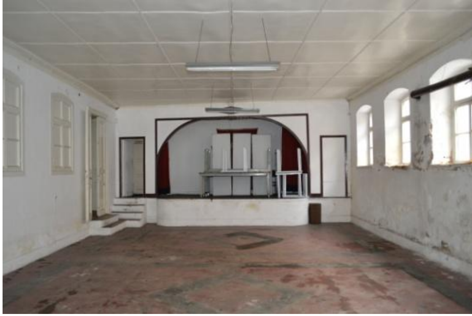
Figure 11: Hall of ceremonies / cafeteria of Kurtuluş R.İ.O. (Author, June 2011).
