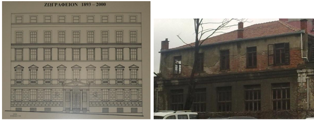
Figure 22: a) Additional floors; Zoğrafyon R.L.İ.O. There are two additional floors on originally three storey high building (Measured drawings, School Panel in Zoğrafyon R.L.i.O., 2000) b) Additional third floor; Merkez R.İ.O.L. Original building height is two storey high (Author, June 2011).
