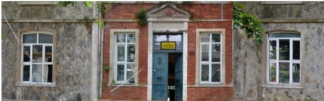
Figure 20: View of front facade, Tarabya R.İ.O., featuring exposed stone masonry on side parts and exposed brick masonry on middle part of the school building.(Author, June 2011).
