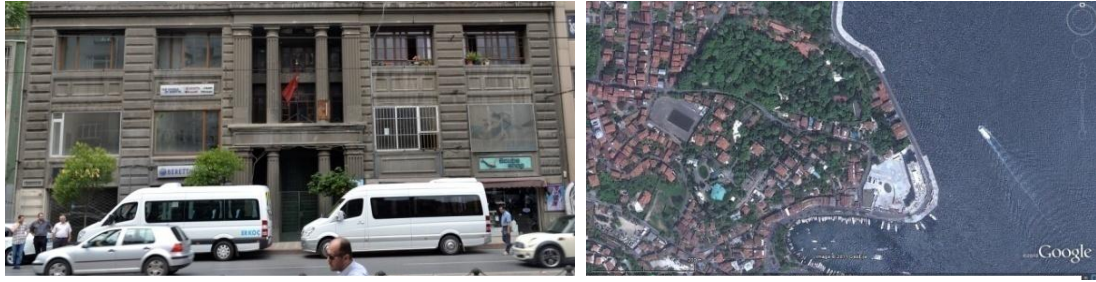
Figure 27: a) Karaköy R.İ.O. is located on Kemeraltı Street, one of Istanbul's commercially most important shafts. b) Tarabya R.İ.O. is in Tarabya, having a good view of the Bosphorus, and eventually located on a valuable parcel (Author, June 2011).
