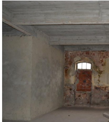
Figure 24: View from new reinforced concrete roofing of Ayakonstantin R.İ.O. (Author, June 2011)
