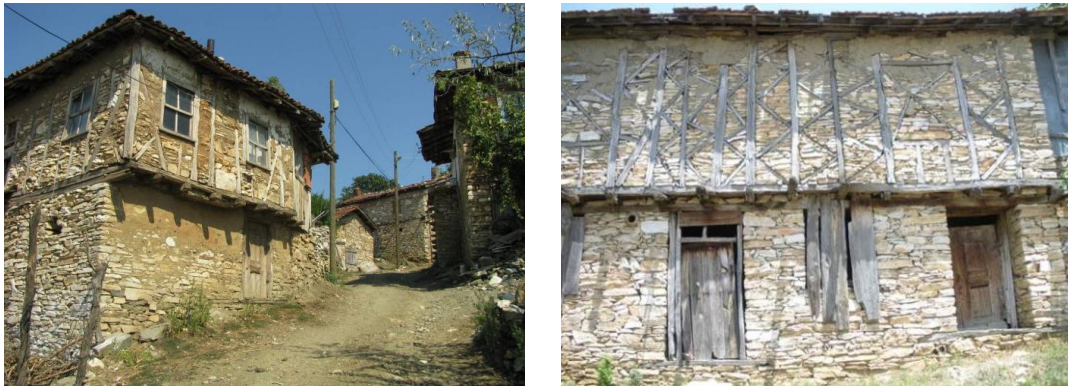
Figure 30. Timber frame construction in traditional houses
