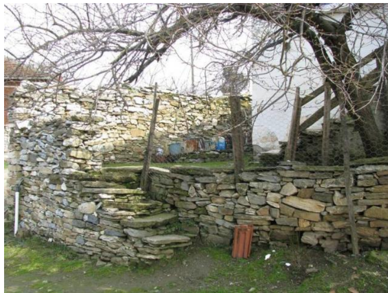
Figure 56. Terraces at the courtyard.
