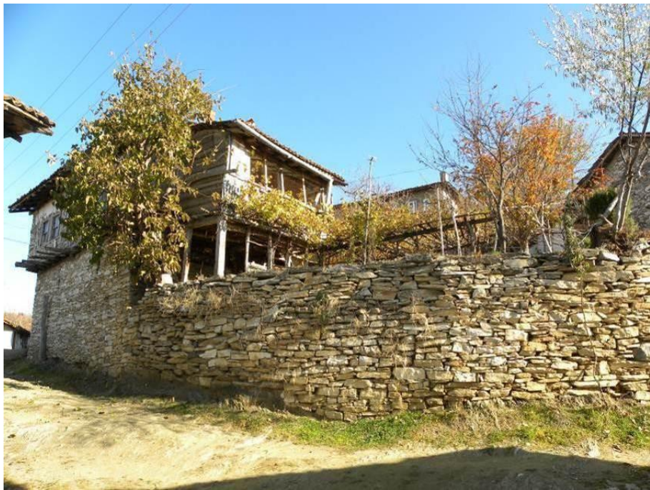
Figure 17. Retaining walls (Photo taken by Fuat Gökçe)
