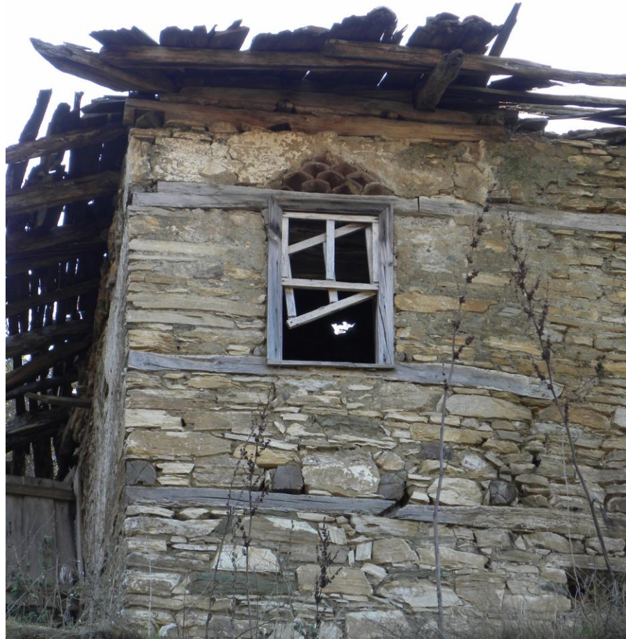
Figure 44. Ornamentations of windows
