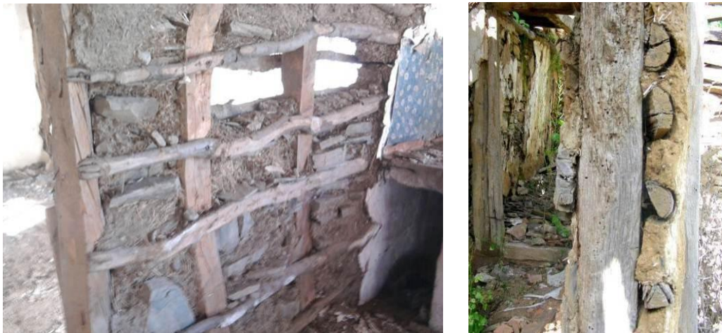
Figure 31. Interior walls with timber frame construction
