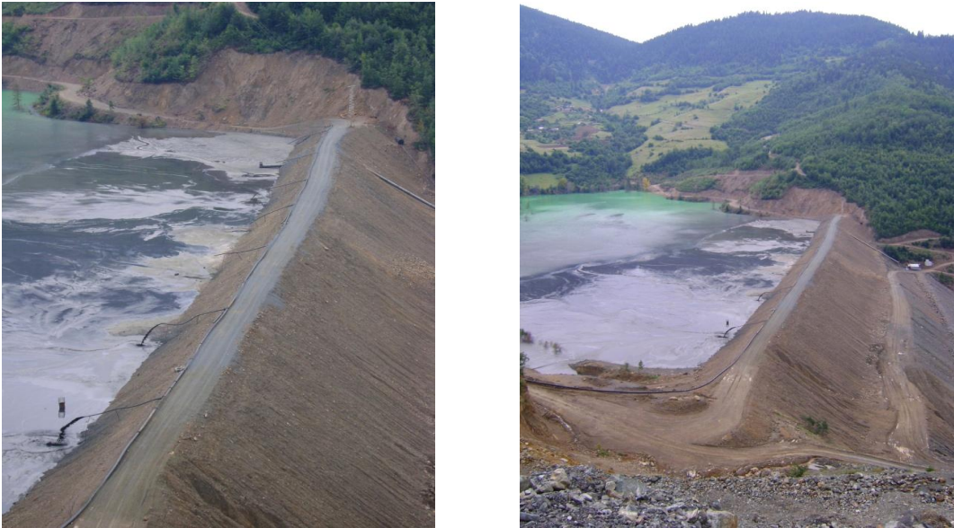
Figure 2.4 Kastamonu Küre copper mine waste storage tailing dam and spigotting process.
