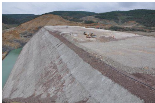
Figure 3.5. Cokal Dam in Construction
