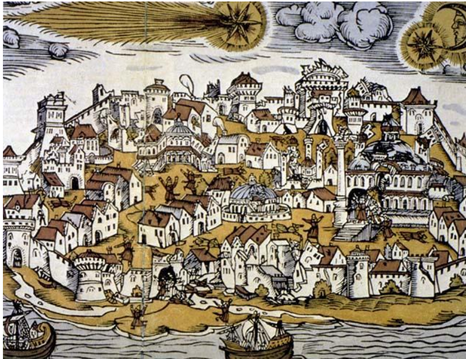
Figure 3.5 Earthquake in Istanbul (March 5th 1556). Hagia Sophia dome and other buildings heavily damaged, many fatalities. Comet was sighted on March 5, 1556 and seen for 12 days. (Nuremberg, 1556). Source: University of California, Berkeley, Pacific Earthquake Engineering Center, Online Archive-Jan Kozak Collection-KZ20
