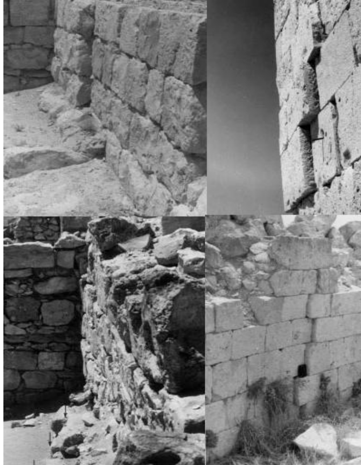
Figure 3.10 City wall's displacements and shifts of individual Stones (A. M. Korjenkov and E.Mazor, 2003)
