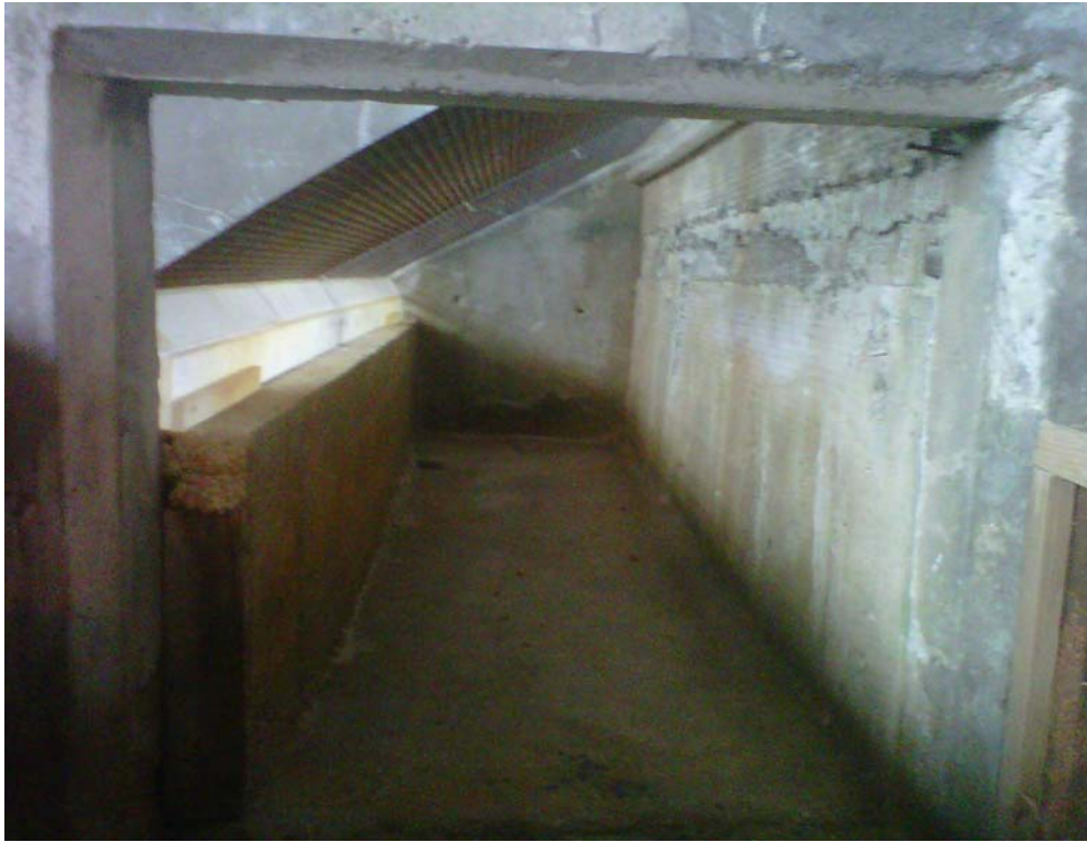
Figure 3.4 Side view of the trash rack and the collection channel
