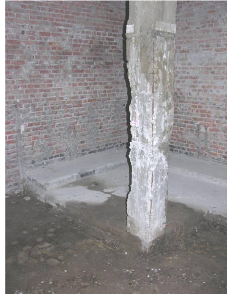
Figure 52 - Fragmentation and corrosion problem of the column (author,2010)
