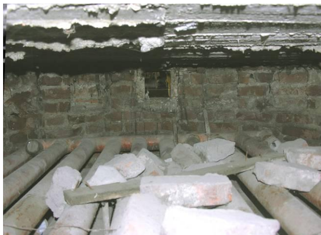
Figure 85– The heating system inside “göbektaşı” (author, 2010)
