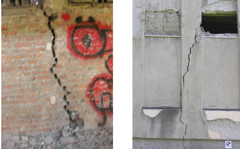
Figure 76 - Structural Crack on east wall both at outer and inner surfaces(author, 2010)
