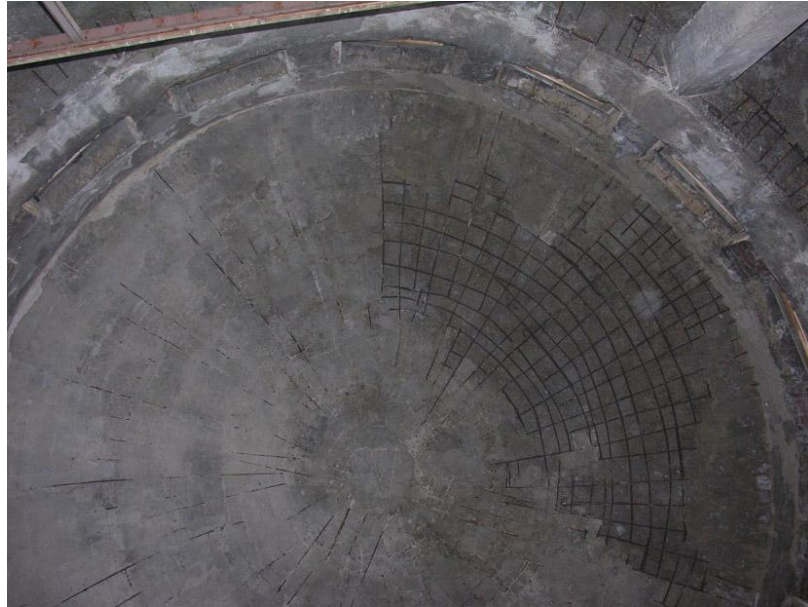
Figure 78 - Concrete fragmentation on dome over space G-01 and F-01(author, 2010)
