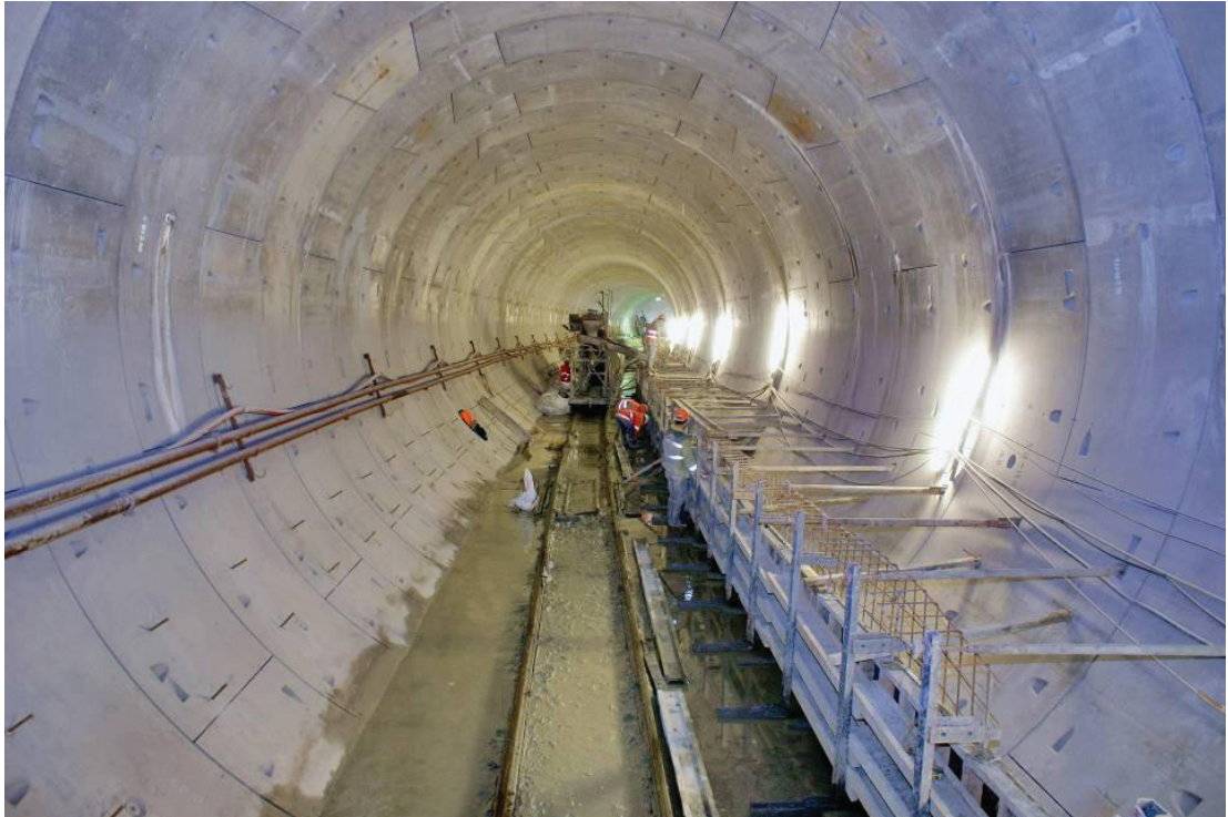
Figure 5.12 A stage from EPB TBM Tunnel Construction
