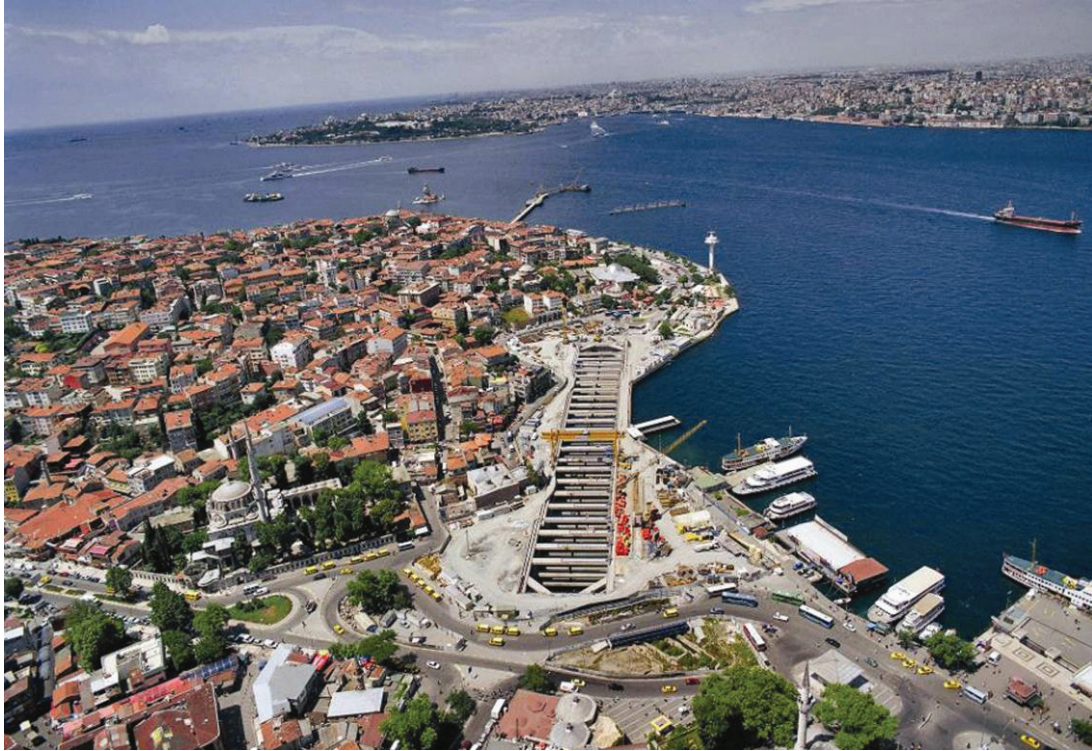
Figure 5.10 A general view of the Üsküdar Station Construction Site
