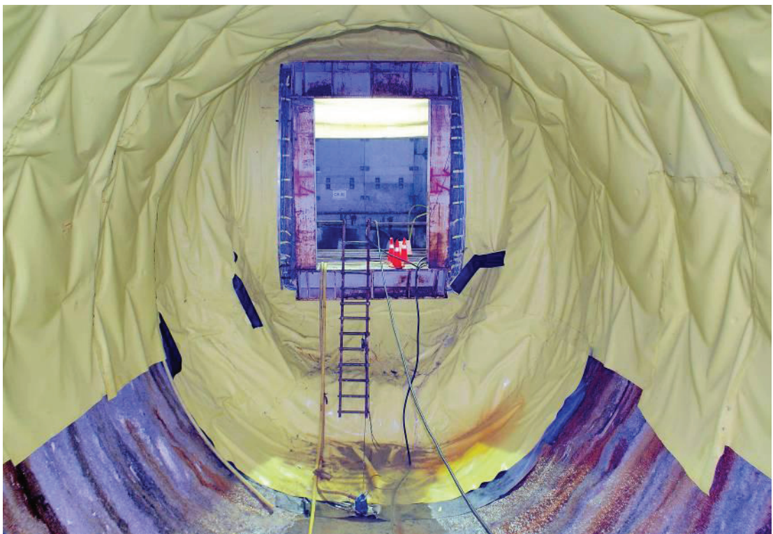
Figure 5.13 A stage from EPB TBM Tunnel Construction
