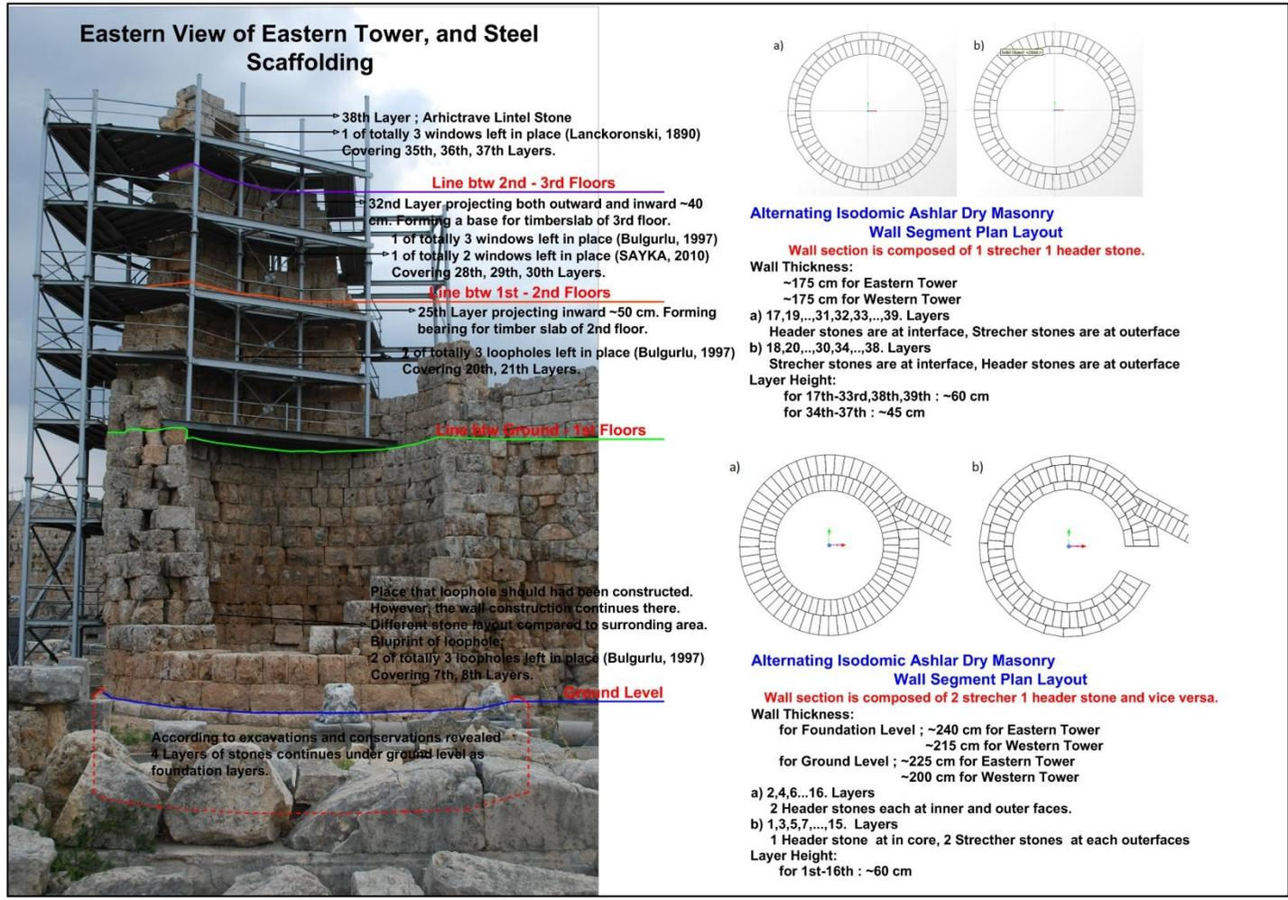
Figure 2.12 Stone Layout Presentation on Eastern View of the Eastern Tower and the Steel Scaffolding
