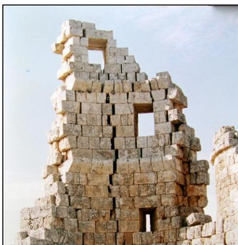
**Figure 2.17** A Vertical Crack at the Eastern Tower Following a Pattern in which Non-Successful Vertical Staggering at Stones exists. Photo by SAYKA (2002)
