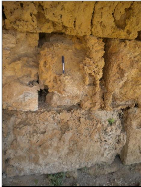
**Figure 2.16** Surface Decay at Lower Levels of the Inner Surface of Tower Walls due to Continuous Wetting Drying Cycles (Topal, 2011).
