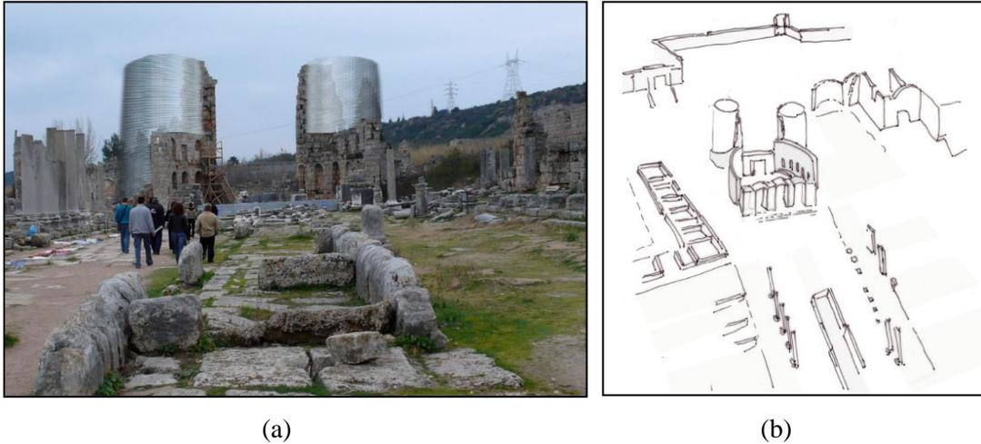
**Figure 4.23** a) The Northern View of Proposed System and Masonry Towers b) Hand Sketch of Hellenistic Propylea and Steel Support Towers (Perbellini, 2010).
