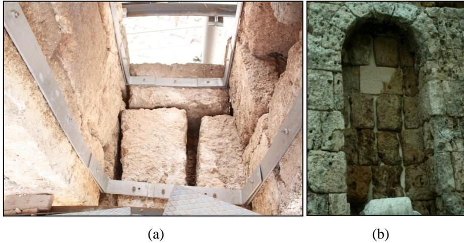
**Figure 2.22** (a) Steel Support Frame Anchored to the Inner Side of 2<sup>nd</sup> Floor Window of the Eastern Tower. (b) Consolidated Part of Courtyard Wall with Filling and Injection (SAYKA, 2009).
