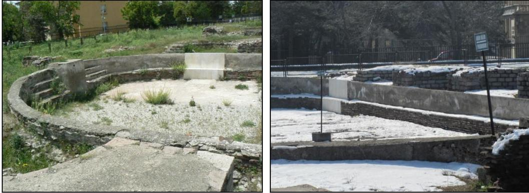
**Figure 62:** The visible deteriorations on the walls of the baths building and the former conservation interventions with cement. (author, 2011)
