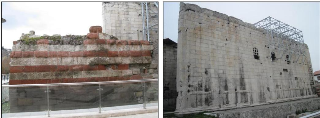
**Figure 52:** Decay forms on the northeast end of the edifice (left) and on the southeast wall of the cella (right) (author January, 2011)
