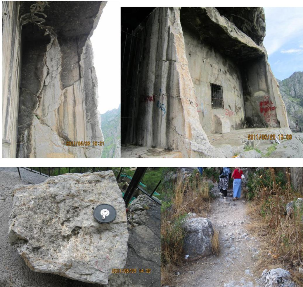
Figure 5.17 Fallen blocks, big failure and hanging blocks on the grave structure
