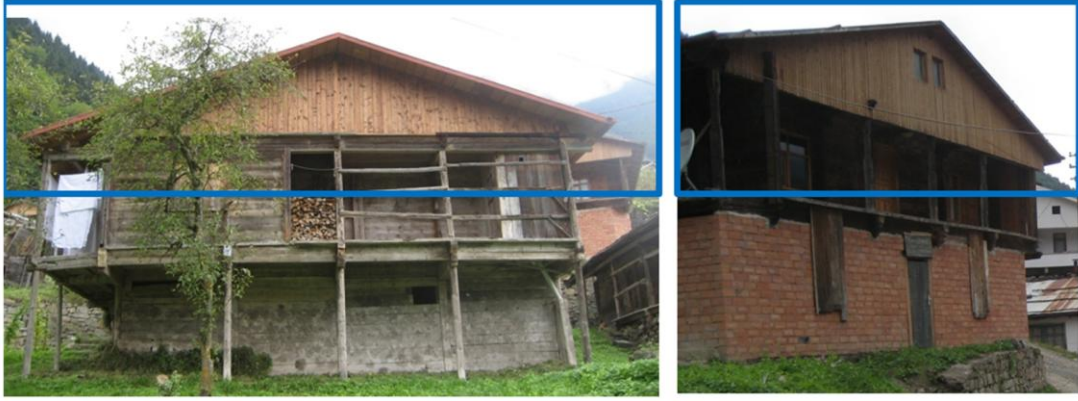
Figure 51, Addition of New Timber Covering to the Triangular Facing of the Roof
