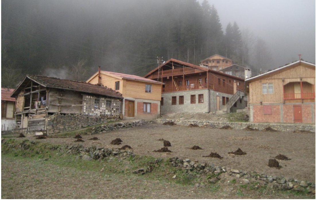
Figure 13, View of the Third Group of Buildings in the Study Area
