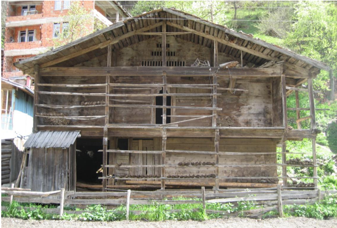
Figure 31, Front Facade of a Vernacular House in Uzungöl
