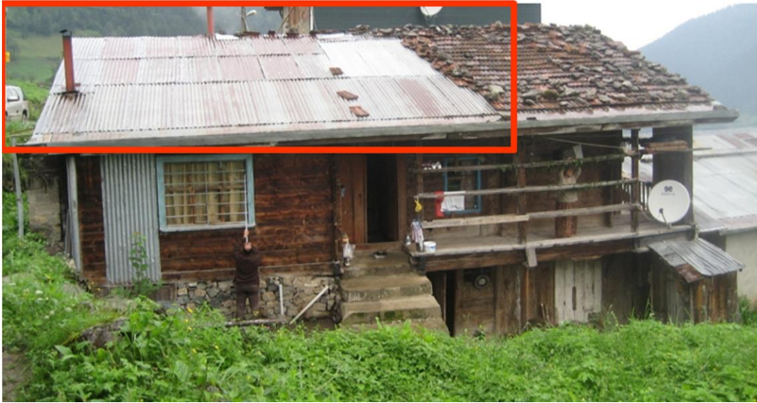
Figure 53, Removal of Some of Roof Tiles
