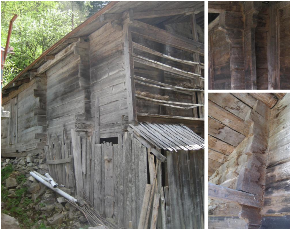
Figure 26, Example of Timber Masonry System Showing the Extension of Walls Towards Outside.
