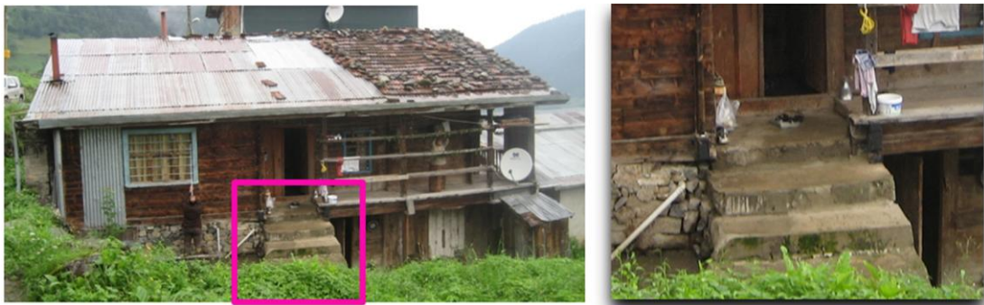
Figure 73, Replacement of the Original Stone Based Stair With Concrete One
