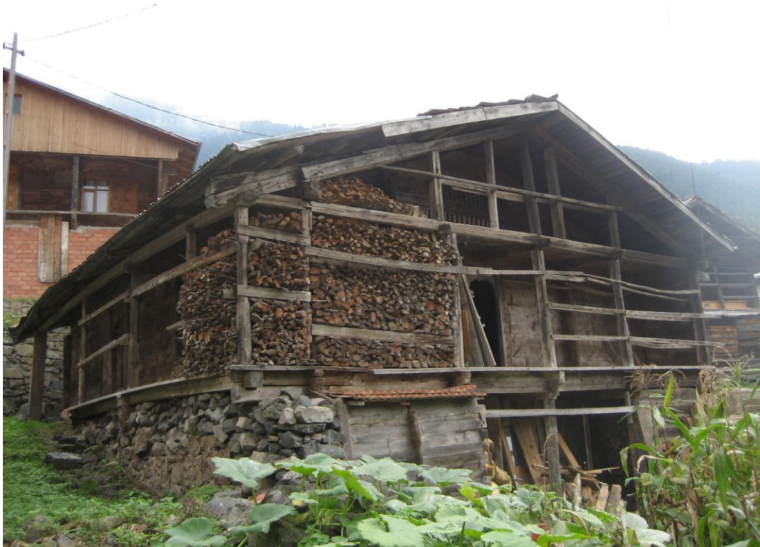
Figure 41, Dış Hayat Placed in Front and Other Open Space on the Side Facade of the Building
