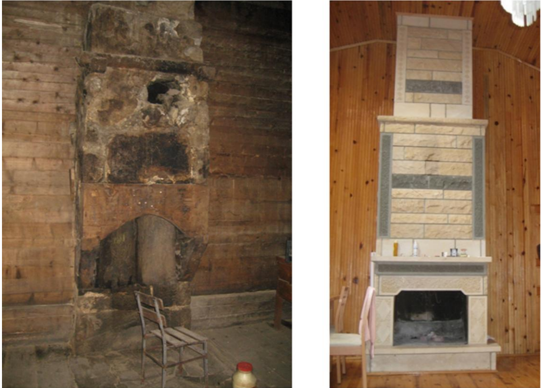
Figure 72, Replacement of the Original Fireplace With New One
