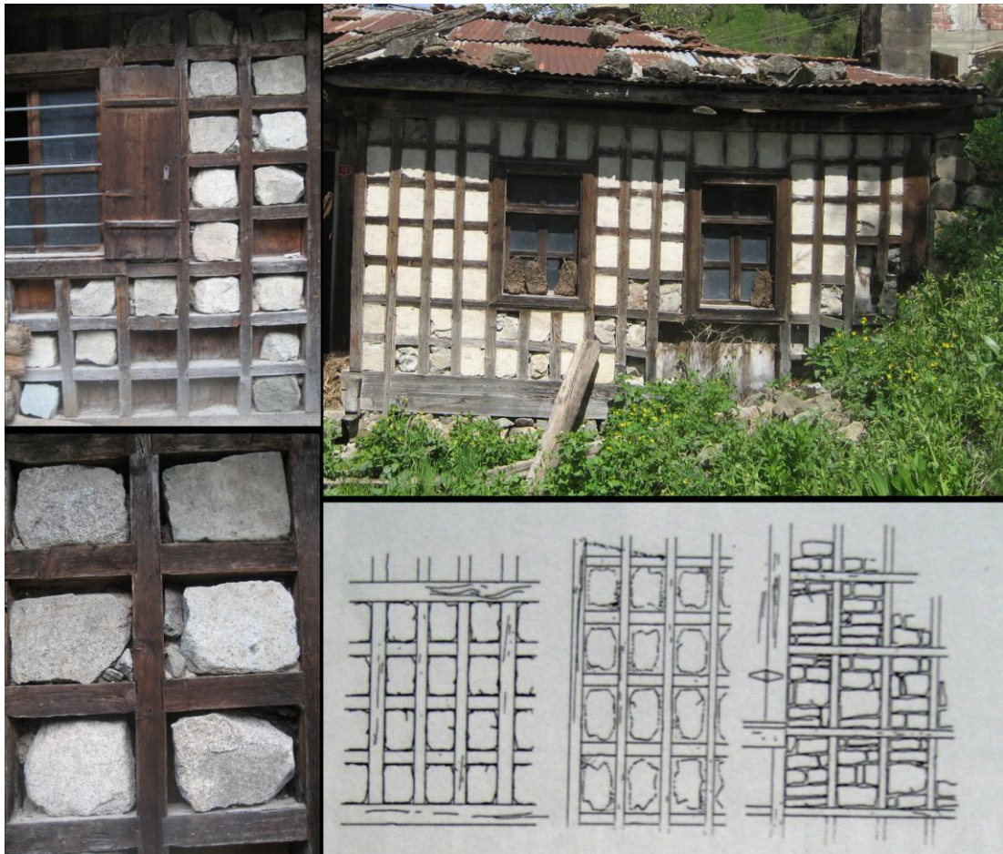
Figure 28, Cellular Type - Göz dolma Construction Technique (Özgüner, 1970: 26)
