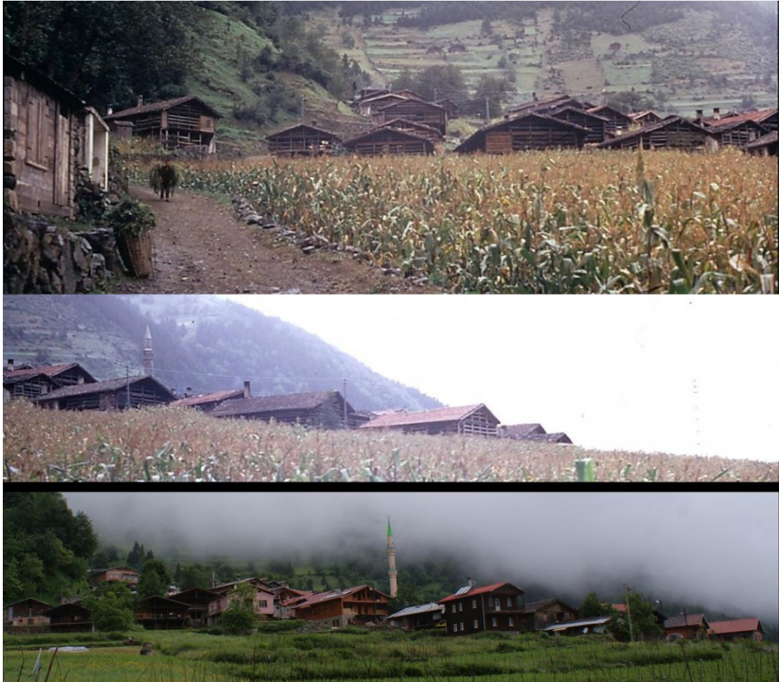
Figure 15, Former and Latter Views of the Study Area. All Houses Have Same Structural System.
