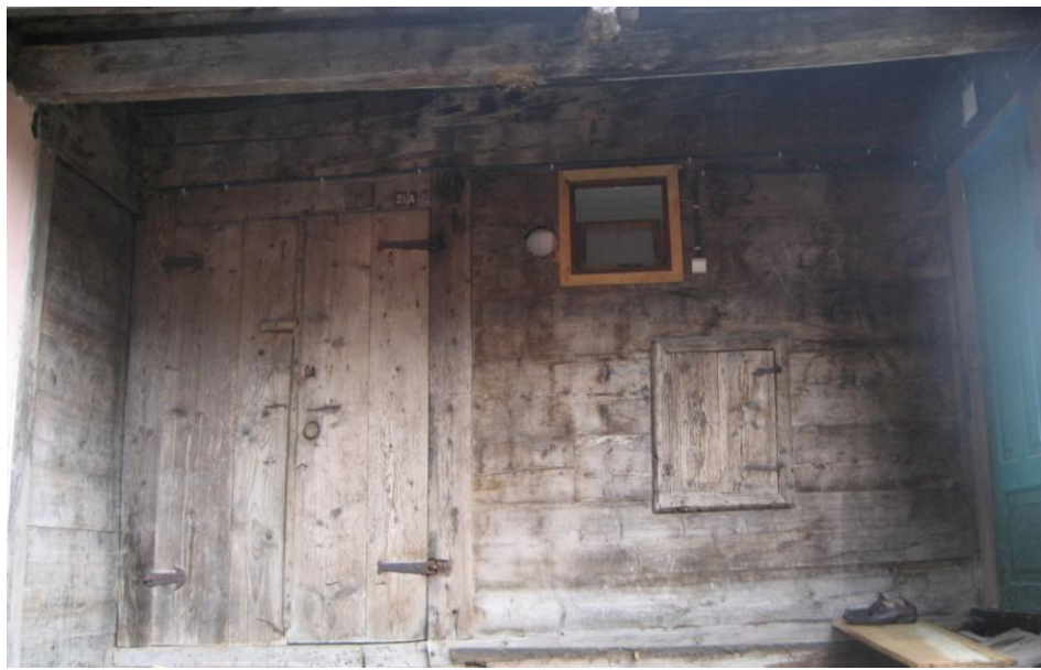
Figure 63, Alteration of Space that Woodshed has been Re-Arranged as Wet Spaces
