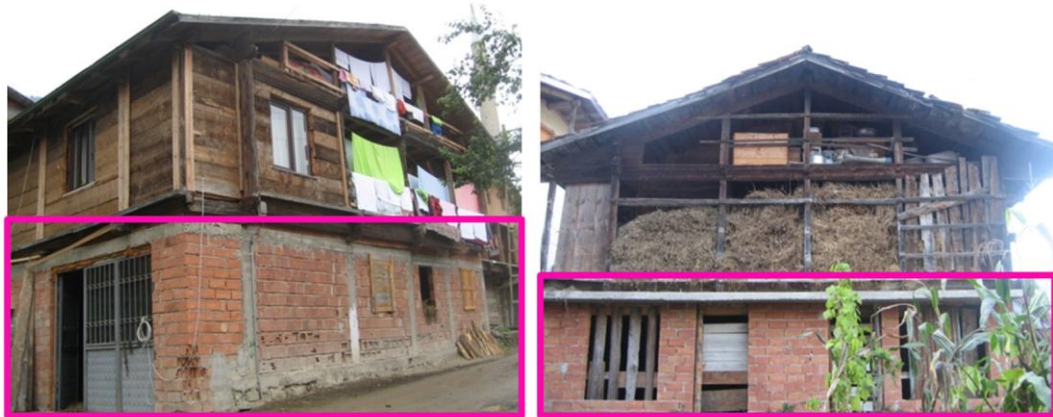
Figure 69, Alteration of the Masonry System of the Basement Floor With Reinforced Concrete System Brick Wall
