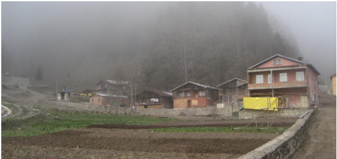
Figure 14, View of the Third Group of Buildings in the Study Area
