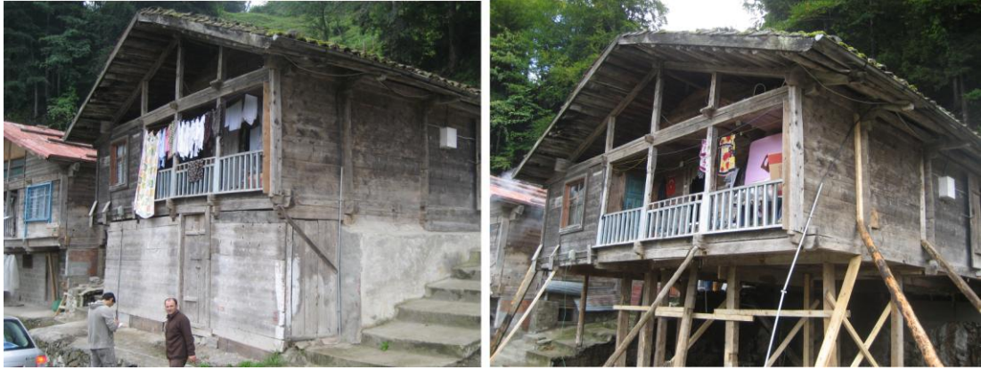
Figure 70, Original View of the House and View During Basement Floor Alteration
