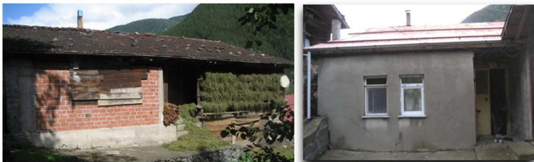
Figure 68, Replacement of the Original Parts of the Building With Reinforced Concrete System Brick Wall
