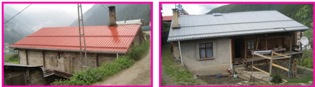
Figure 71, Renewal of the Roof With New Material
