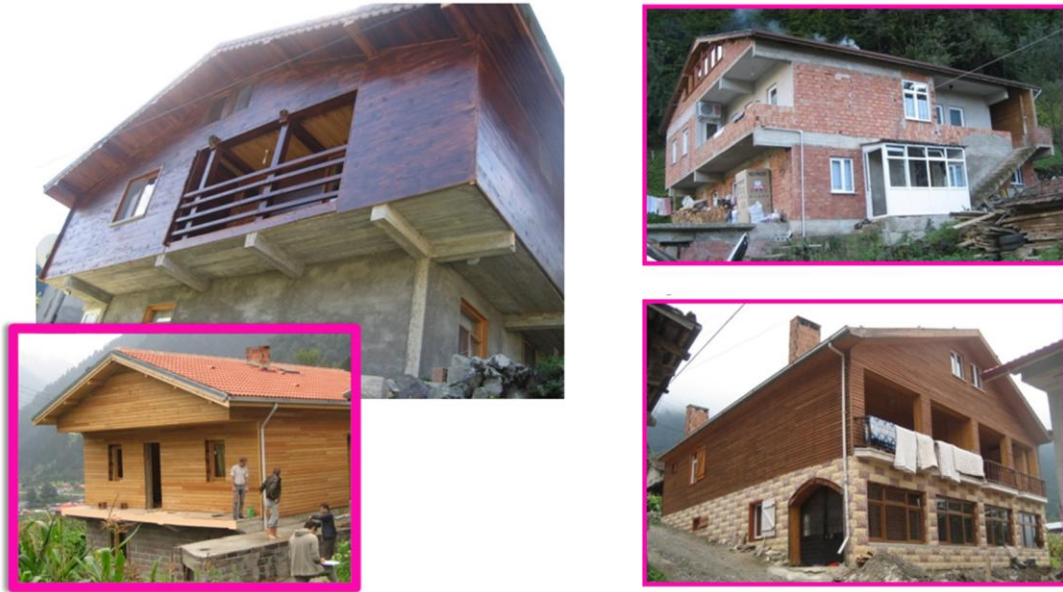
Figure 54, Alteration of Whole Building
