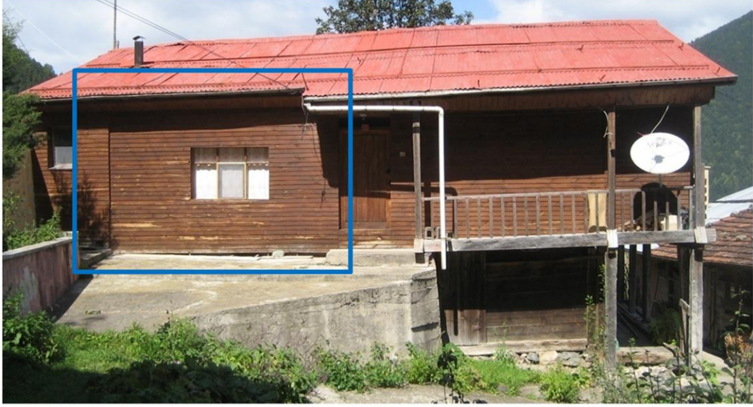
Figure 50, Addition of New Timber Covering to the Façade
