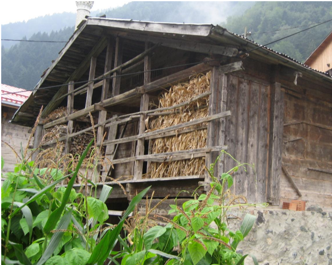
Figure 34, Gable Roof of a Vernacular House in the Study Area
