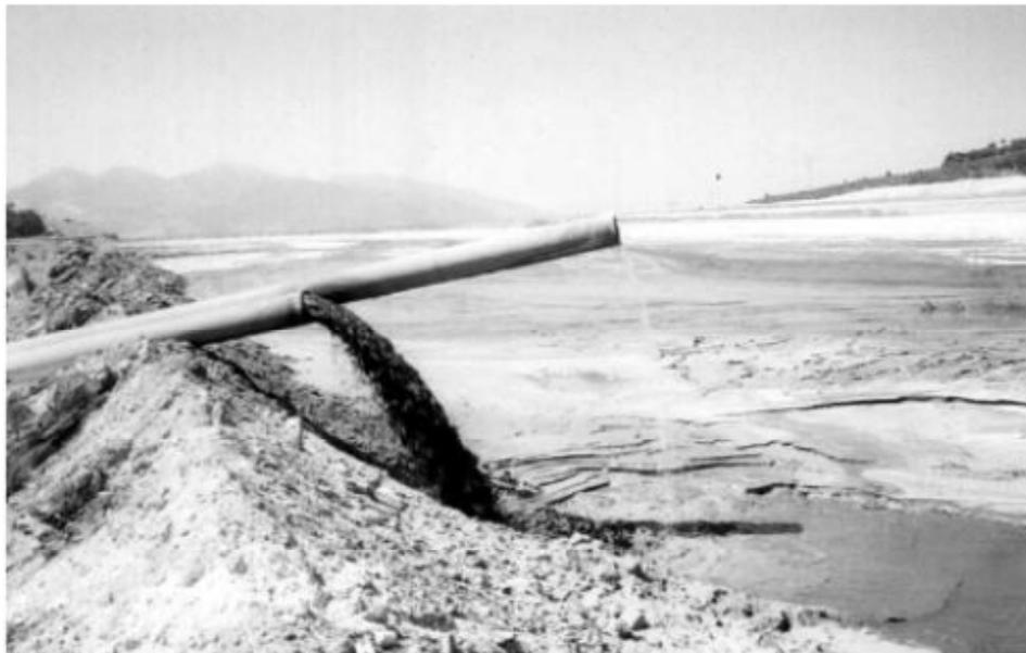
Figure 3.2 Ash Disposal Site of Soma Thermal Power Plant
