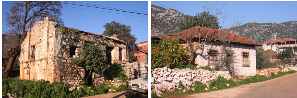
Figure 68. Çevreli village, examples of vernacular architecture (February, 2011)
