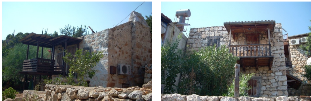
Figure 74. Kaleköy, examples of vernacular architecture (May, 2010)
