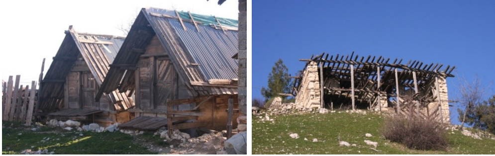
Figure 79. Timber granaries and abandoned house in Çataloluk village (February, 2011)
