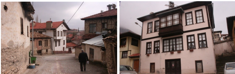
Figure 82. Traditional houses in Elmalı (February, 2011)
