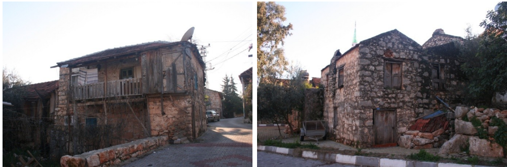
Figure 70. Üçağız village, examples of vernacular architecture (May, 2010)
