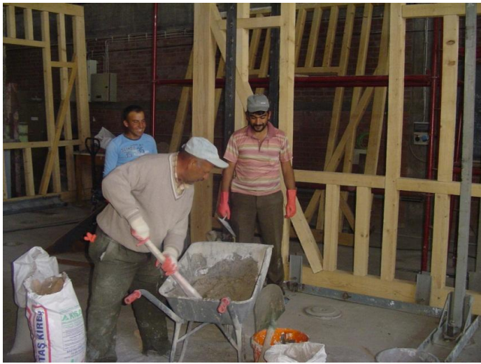
Figure 137: Preparation of mortar for the infill
