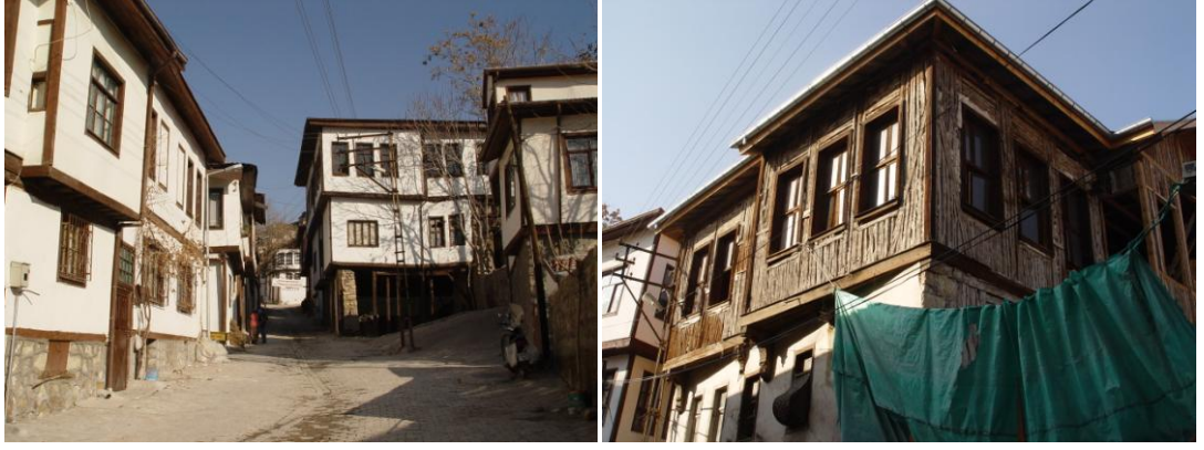
Figure 3: Traditional Beypazarı houses (Neriman Şahin Güçhan archive)
