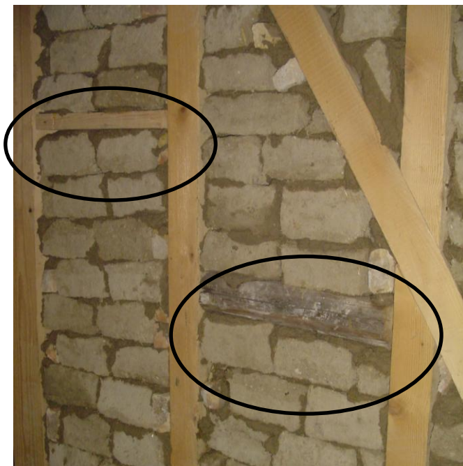
Figure 84: Addition of hatils between existing timber elements
