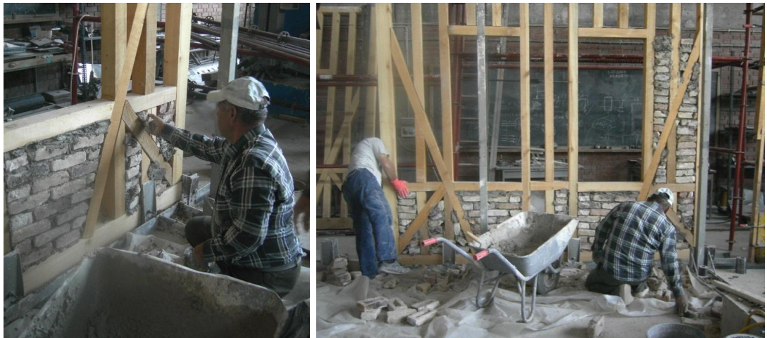
Figure 107: Infilling process
