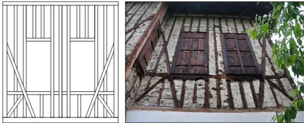
Figure 46: Frame module with two window openings from Akpınar St. No: 20, Karaali District, Safranbolu
