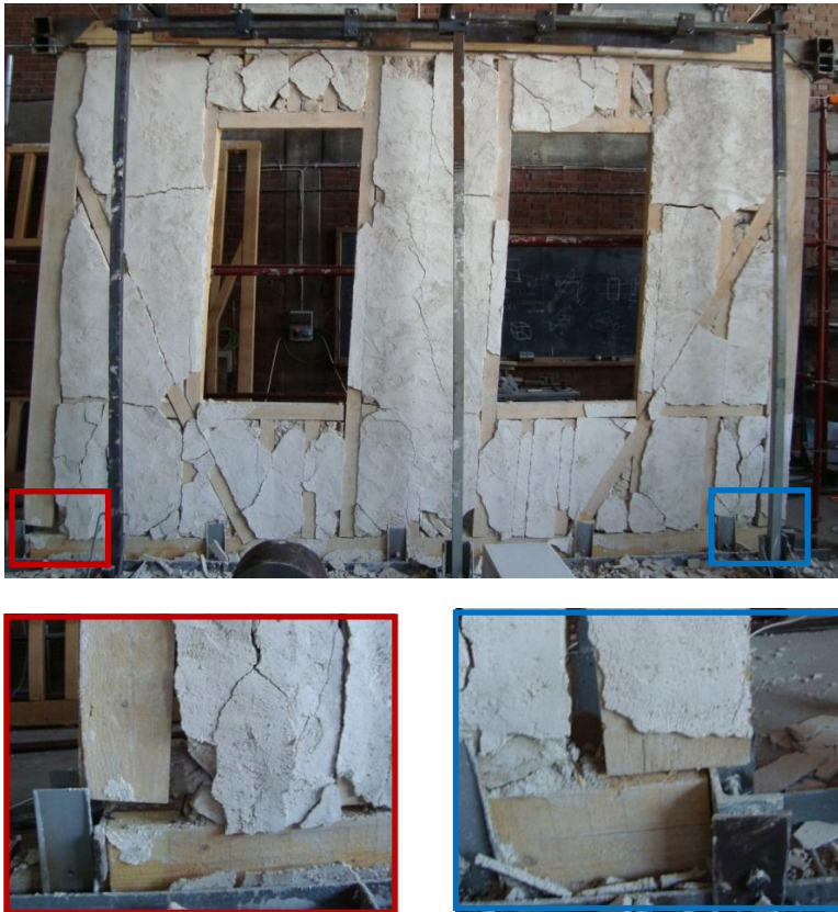
Figure 143: Frame#7 with infill after the test
