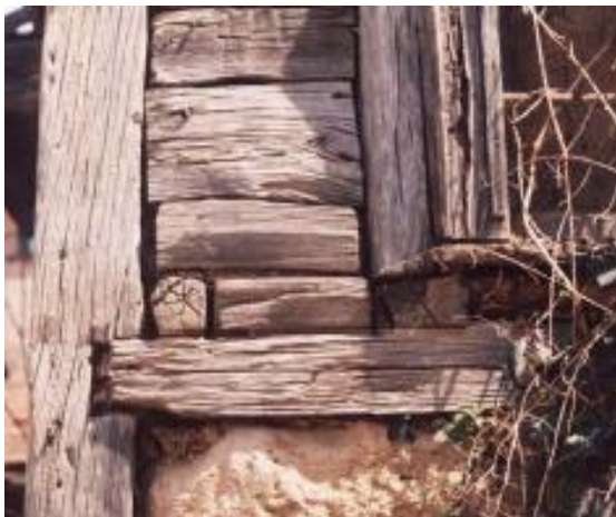
Figure 30: Upright element – horizontal element connection of a house in Yukarı Değirmendere (Aksoy and Ahunbay; 2005)
