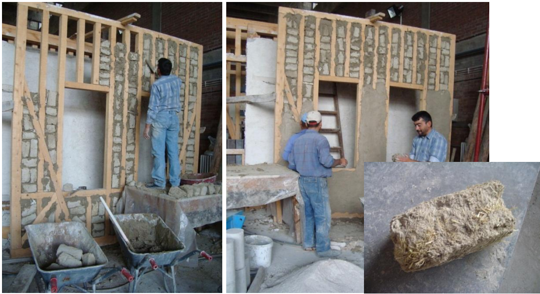
Figure 72: Infilling and plastering processes
