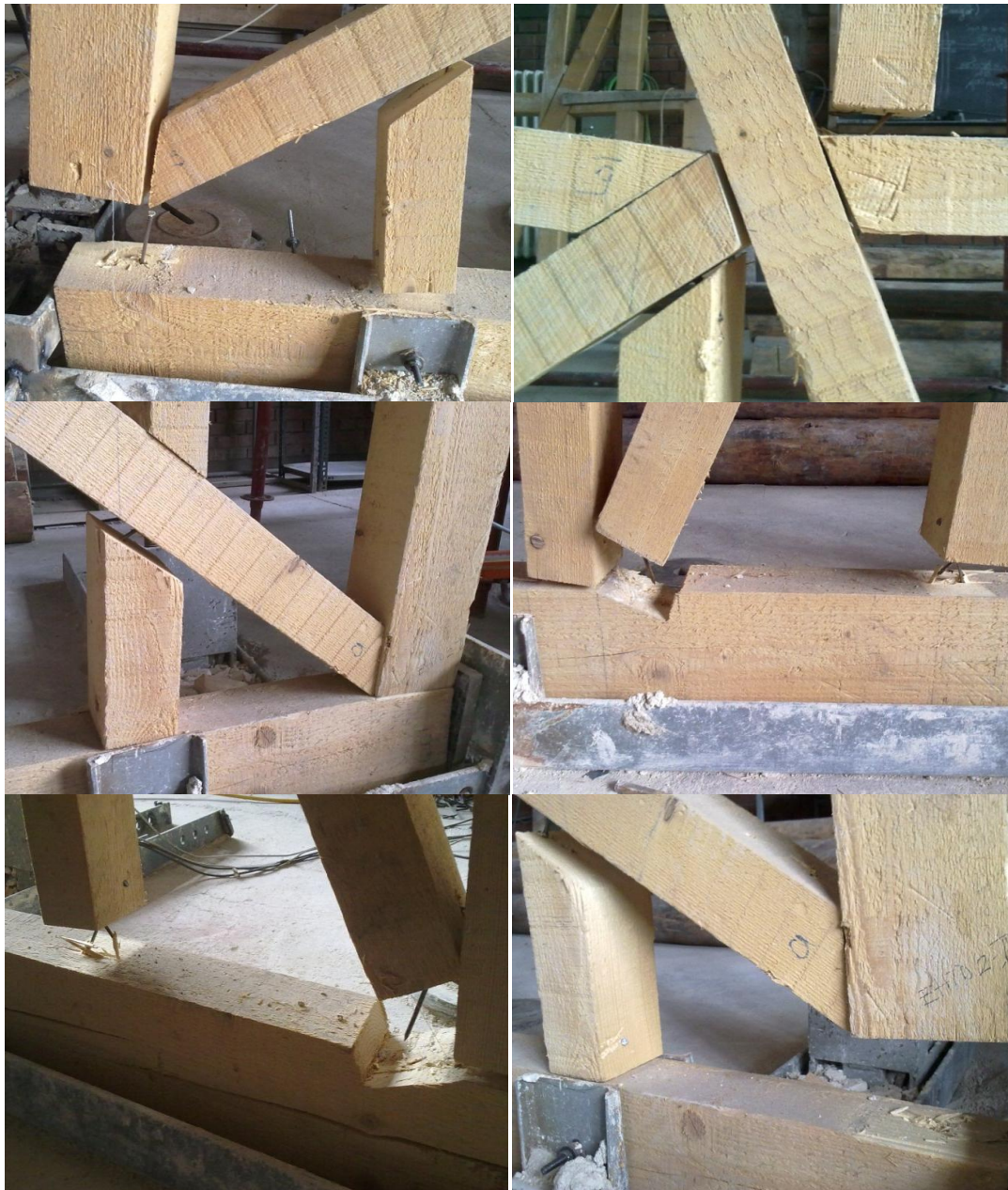
Figure 151: Examples to connection dilatations observed during the testing of Frame#8
