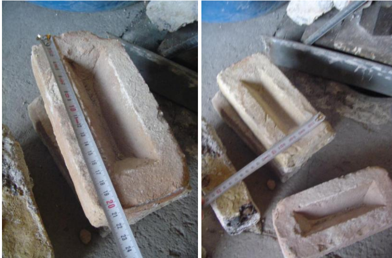
Figure 106: Solid bricks used for infill
