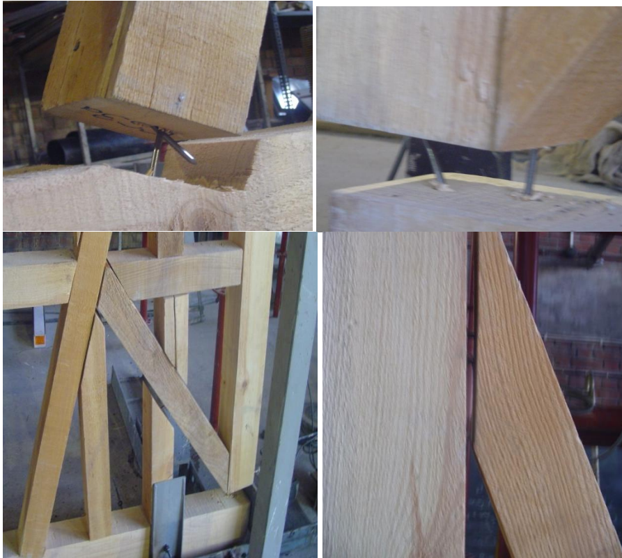
Figure 105: Details of dislocated connections observed during the testing of Frame#4
