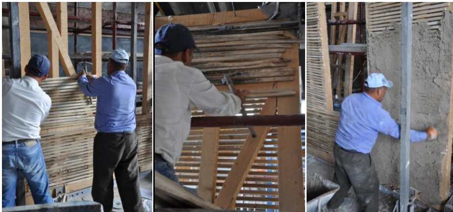
Figure 153: Bağdadi covering and plastering
