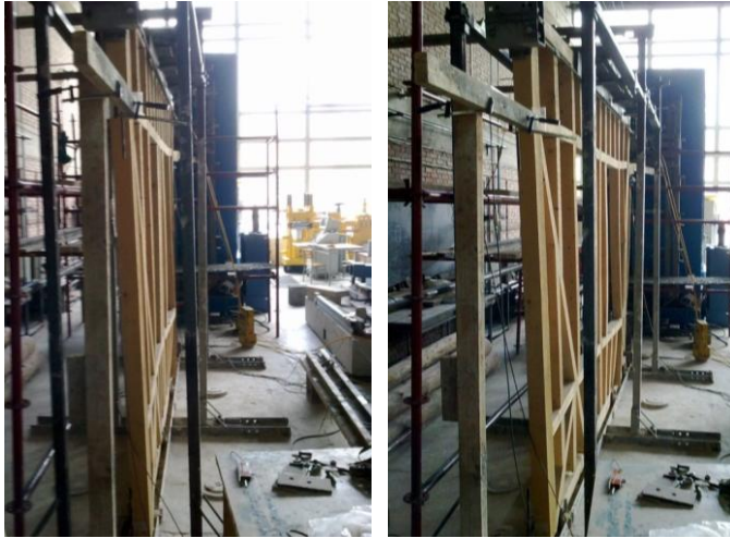
Figure 152: Overall permanent out-of-plane displacement after the testing of Frame#8
