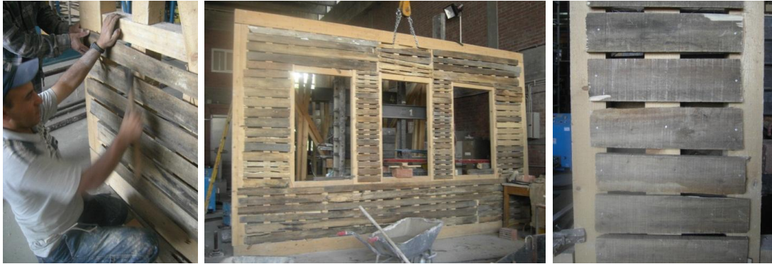
Figure 127: Nailing of laths
