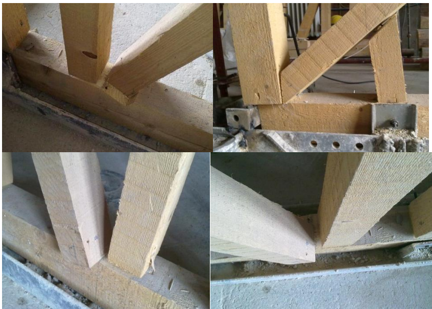
Figure 150: Examples to out-of-plane displacements occurred at the connections after the testing of Frame#8
