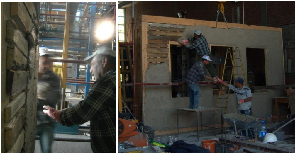
Figure 128: Plastering process
