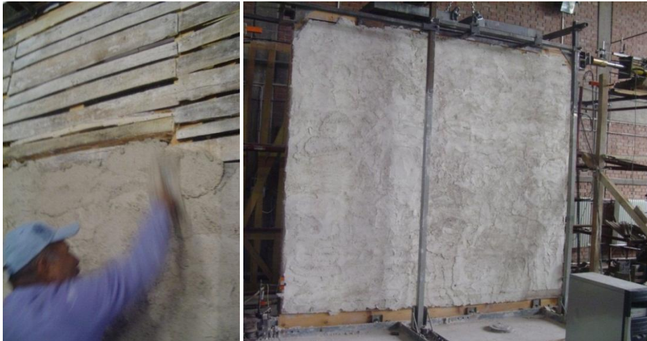
Figure 96: Plastering and the final state of the Frame#3 with şamdolma covering
