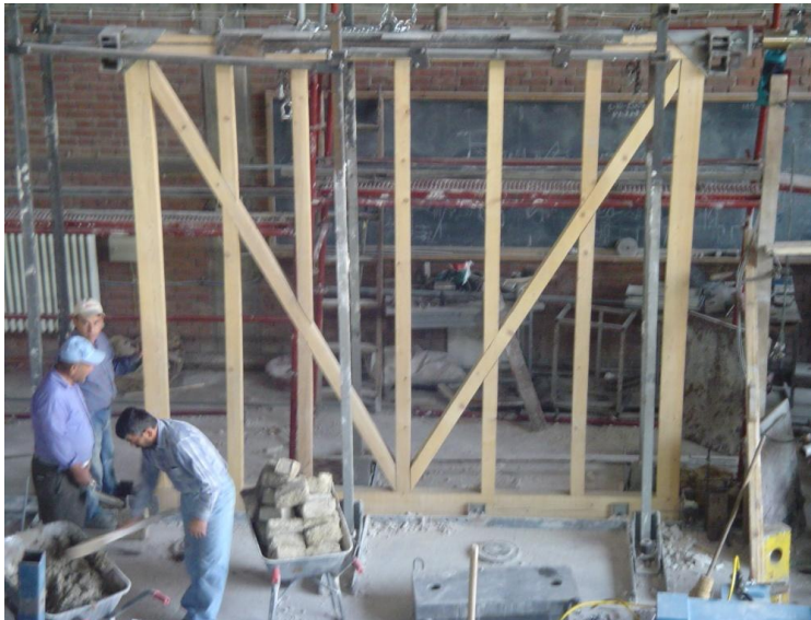
Figure 82: Frame#2 after repairing all connections
