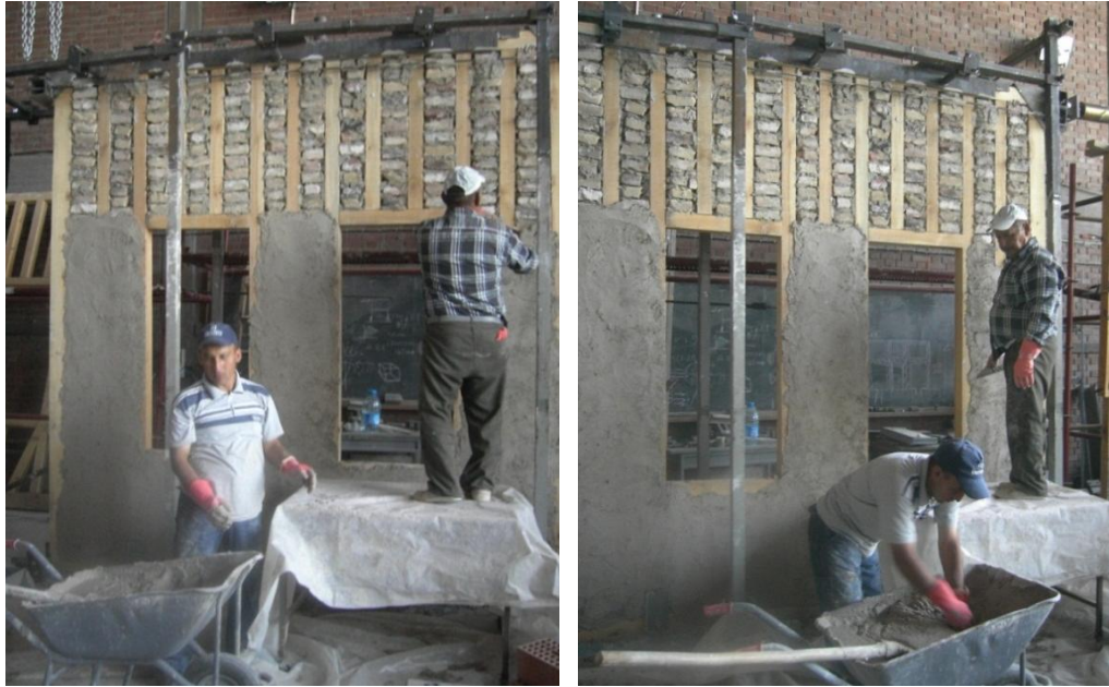
Figure 108: Plastering of Frame#4 with brick infill
