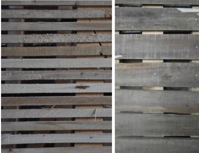
Figure 41: Bağdadi and şamdolma covering techniques, respectively
