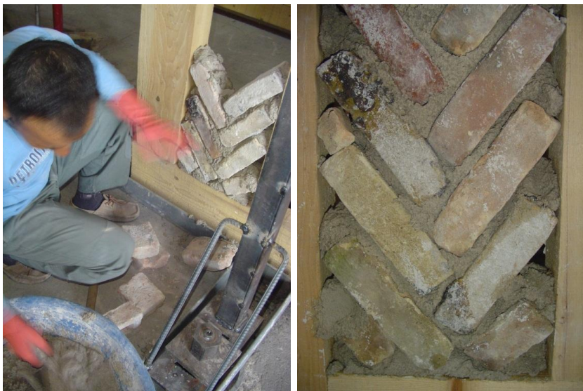
Figure 138: The infill was laid in the herring bond style
