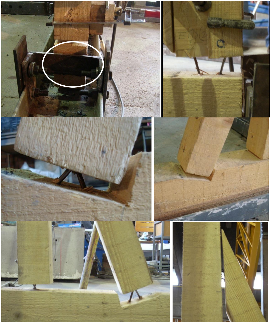
Figure 70: Several examples to joint failure in the testing of Frame#1
