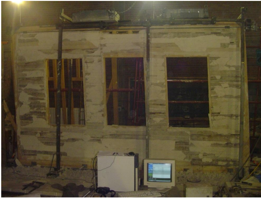
Figure 131: Frame#6 with infill after the test
