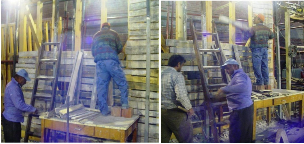
Figure 95: Nailing of laths
