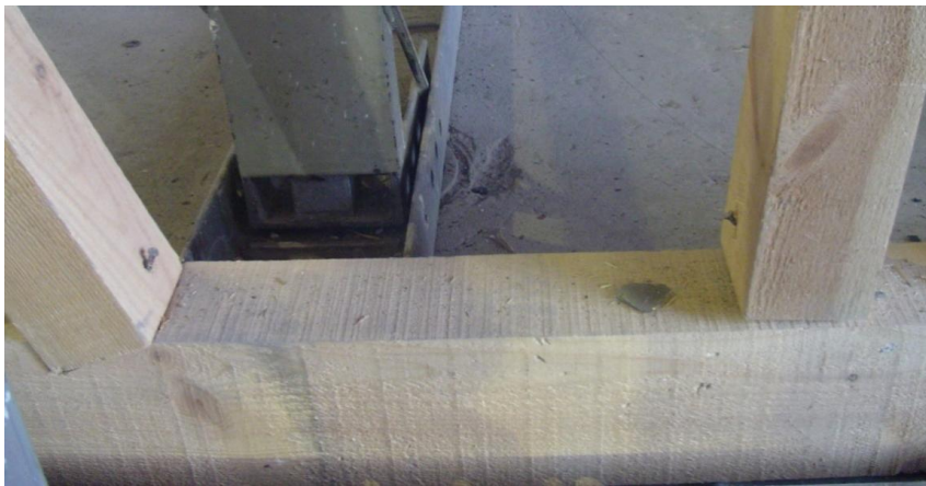
Figure 104: Permanently dislocated nails during Test#4
