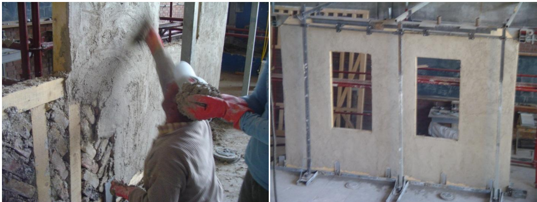
Figure 140: Plastering and the final state of the Frame#7 with infill
