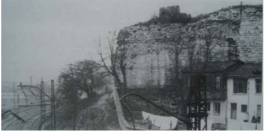
Figure 12 Demolition of wall during the construction of railway
