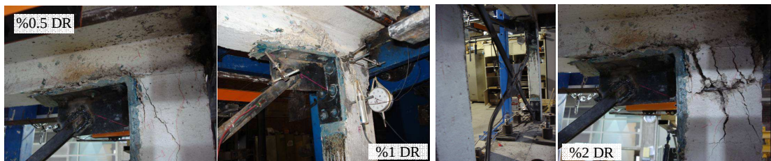
Figure 2.53 Picture of the X-Braced frame damage
