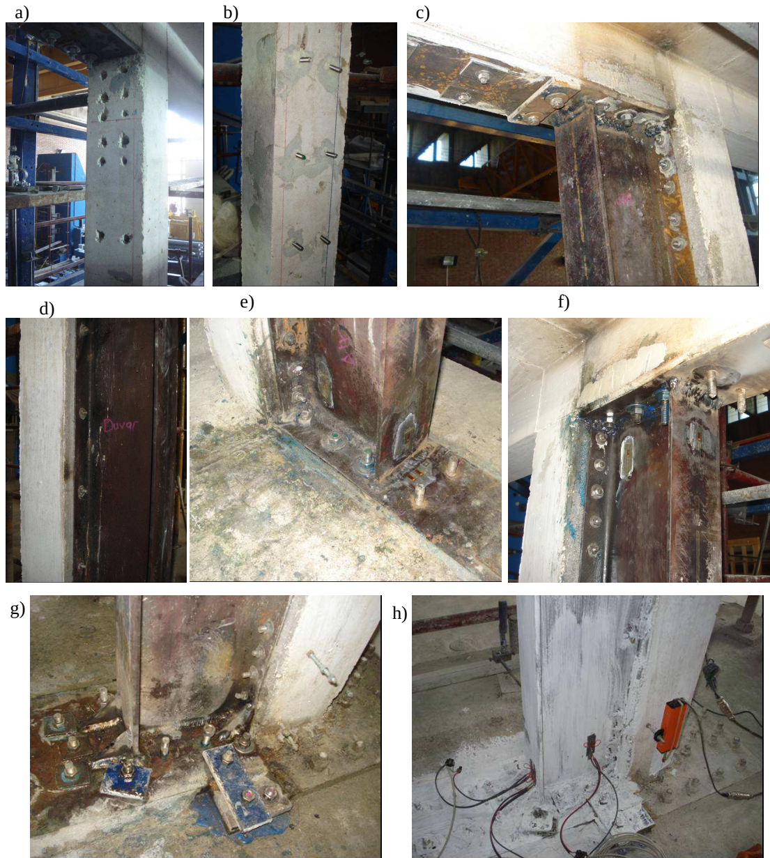
a) 2 story top of the bottom of column, b) 2. story column, c) 2 story joint, d) 1story column, e) 2 story bottom of the column (1. story joint), f) 1 story top of the column (1. story joint), g and h) 1 story bottom of the column or connection at the base.
