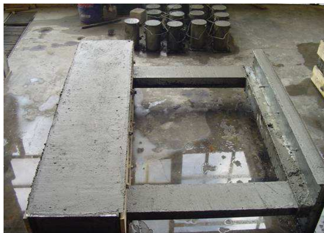
Figure A1.4 RC frame after concrete casting
