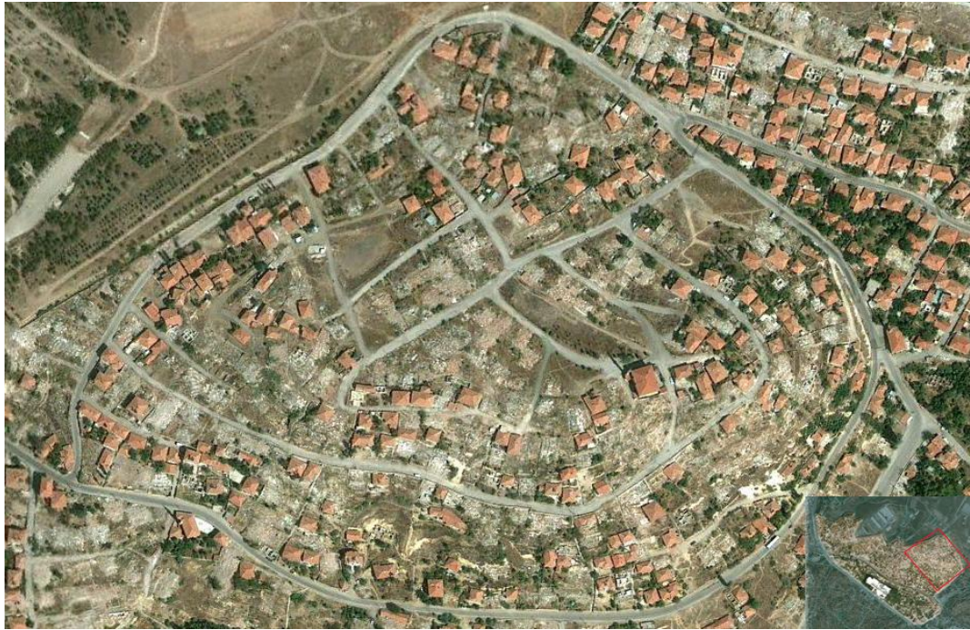
Figure 4.27. Derbent Neighbourhood's Aerial Photograph (Demolished and Not Demolished Areas at Northeast) (Source: Google Earth (prepared by author)).
