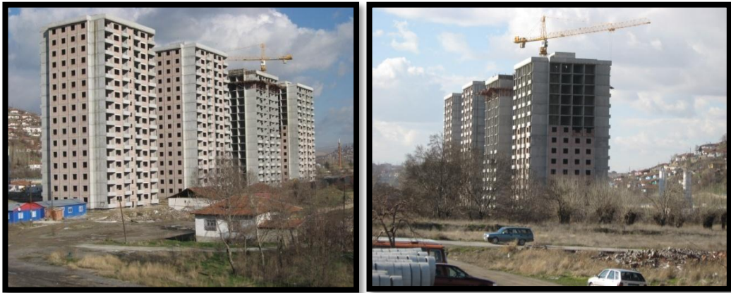
Figure 3.20. First Stage Constructions in Derbent ( Source: Great Municipality of Ankara New Mamak UTP Coordination Centre)
