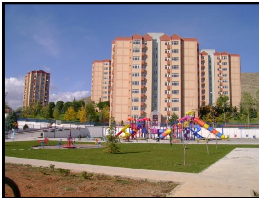
Figure 3.18. A view from Eserkent Mass Housing Area (Source: Personal Archive)
