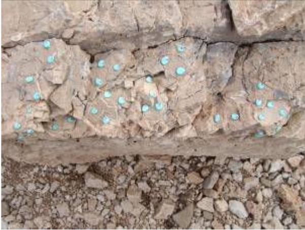
**Figure 3.55** View of Nemrut limestone treated with nanodispersive  $\text{Ca(OH)}_2$  solution
