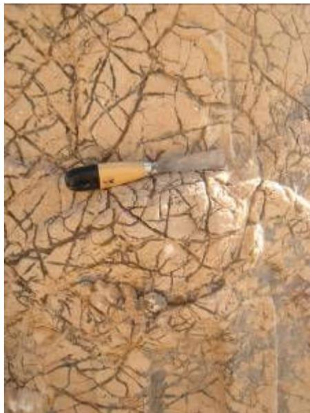
**Figure 3.2** View of fragmental disintegration through cracks filled with biological deposition on one of the Nemrut Dağ Monument statues (West terrace, a detail on the head of Herakles).
