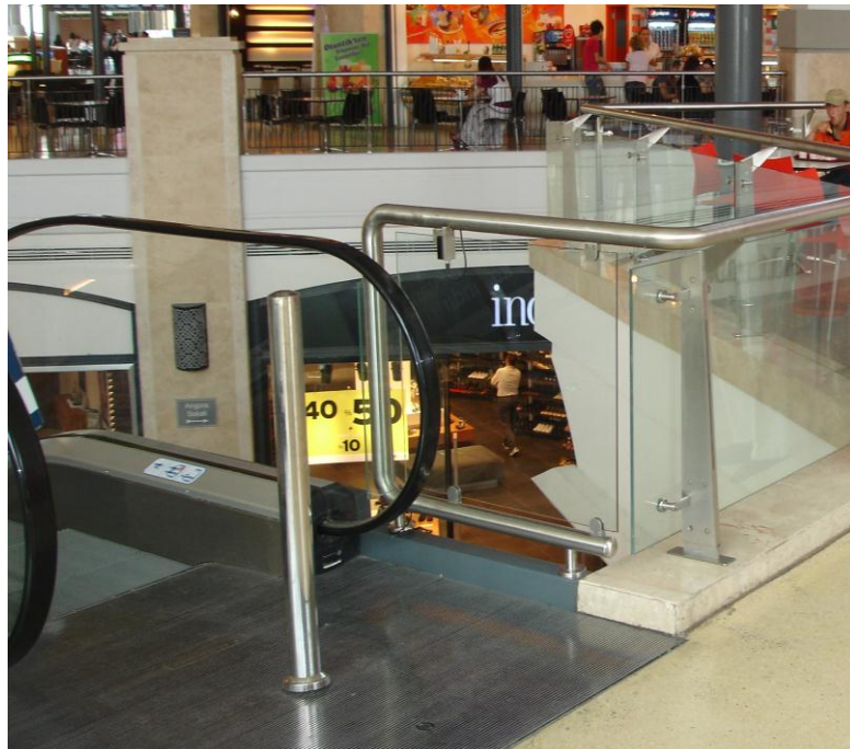
Figure 76. Detail showing the parapet finishing at the corner together with the safety measures.
