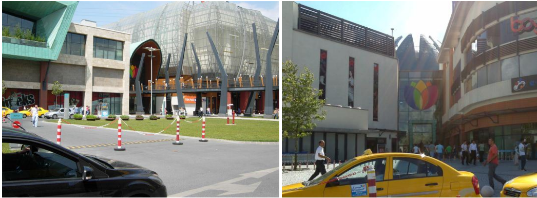
Figure 64. South and North-east Entrances of Forum Istanbul, at different Ground Levels.
