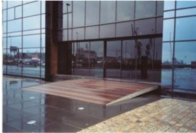
Figure 53. This entrance is virtually impossible to distinguish from adjacent window panels. (Giuliani, 2001)
