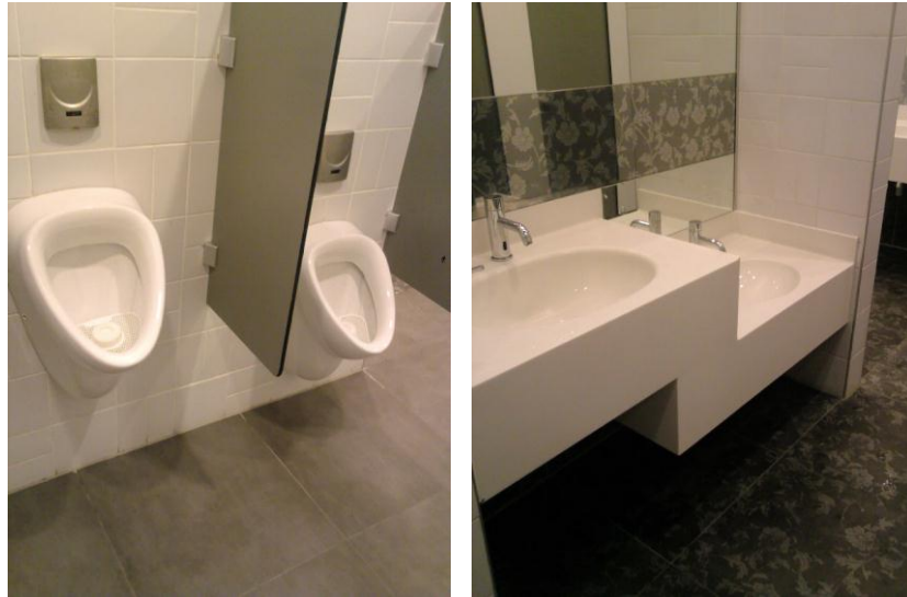
Figure 86. The urinals different heights and the lavatory's two counter heights and motion activated faucets provide accommodations that are usable by a wide range of users in the typical restrooms of Forum Istanbul.
