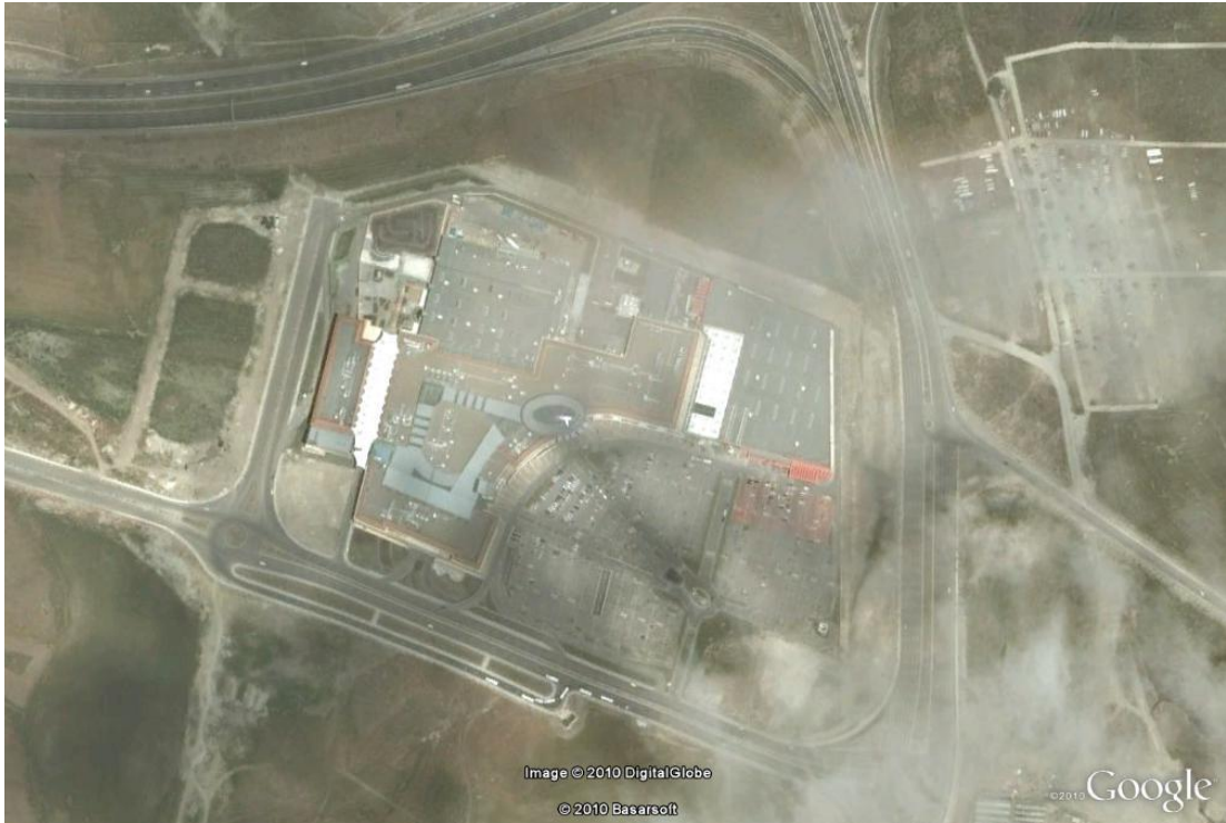
Figure 28. Aerial View of Forum Ankara Shopping Center. Google Earth Image, retrieved on June, 2010.
