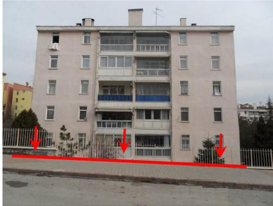
Figure 7.18. A building facade image, in which the height difference between the building baseline and the pavement is evident.
