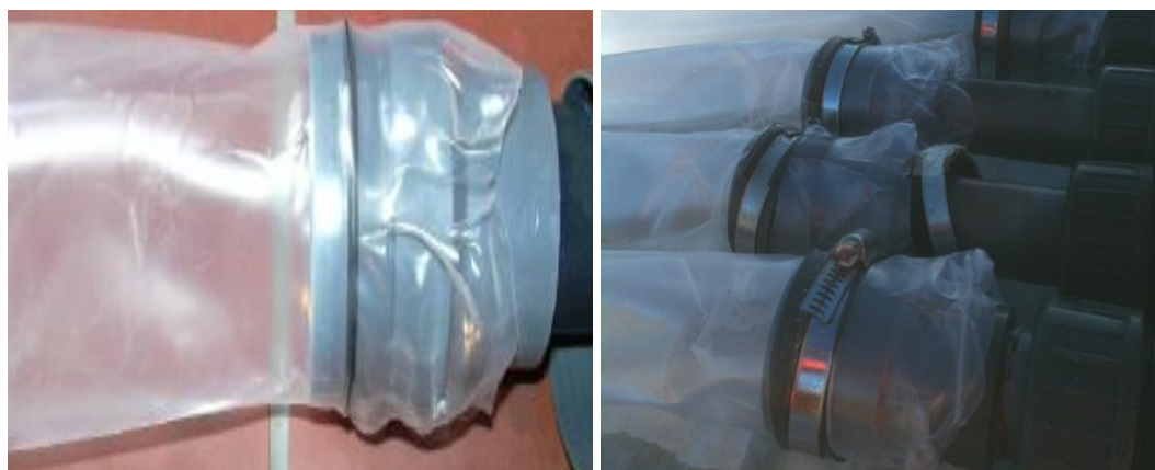
Figure 3-9 The installation of the LDPE tubes to the manifold
