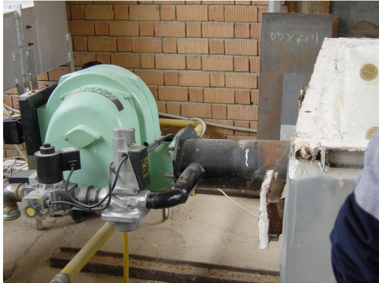
Figure 3.9 Alarco Lamborghini Natural Gas Burner
