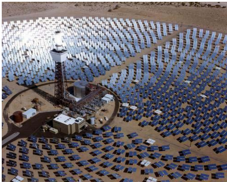
Figure 1.3 Power Tower System [9]
