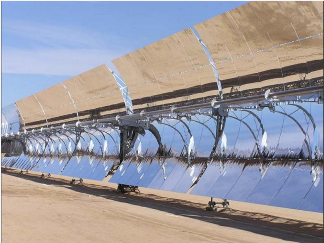
Figure 2.1 Solar Collector Assembly
