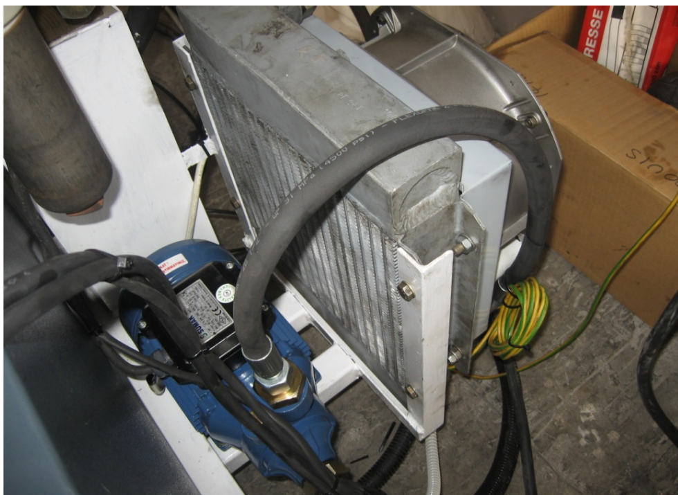
Figure 4.8 – A view of hydraulic power pack oil cooler
