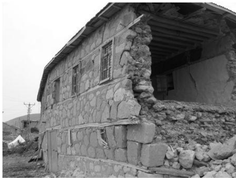
Figure 4. 15. Examples of masonry dwellings damaged during the 2010 Elazığ earthquake with out-of-plane failure of exterior walls (photos taken by the METU-EERC team)
