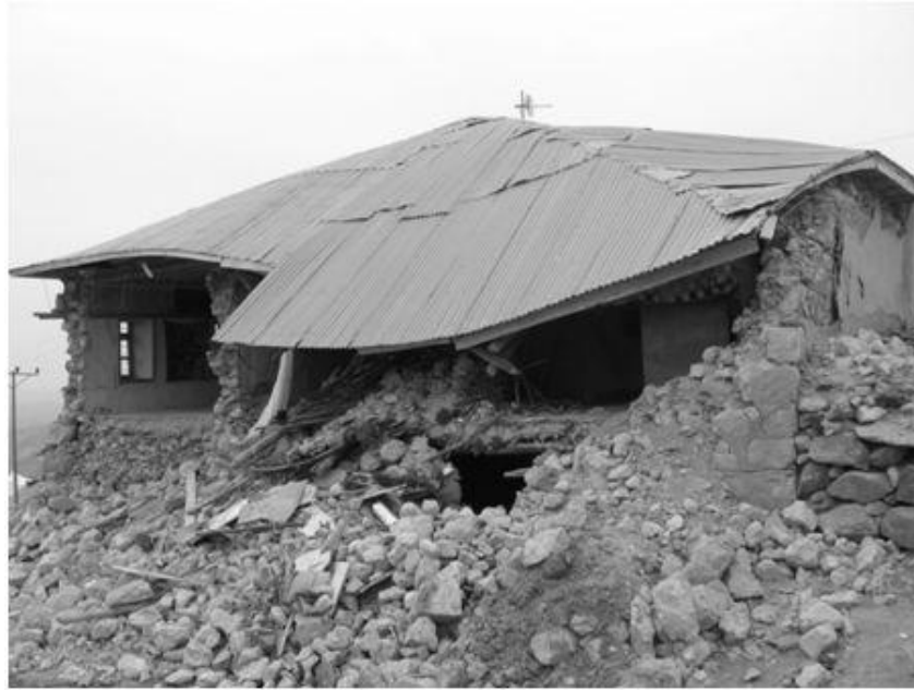
Figure 4. 16. Poor wall-to-wall and floor-to-wall connections leading to out-of-plane type of damage during the 2010 Elazığ earthquake (photo taken by the METU-EERC team)
