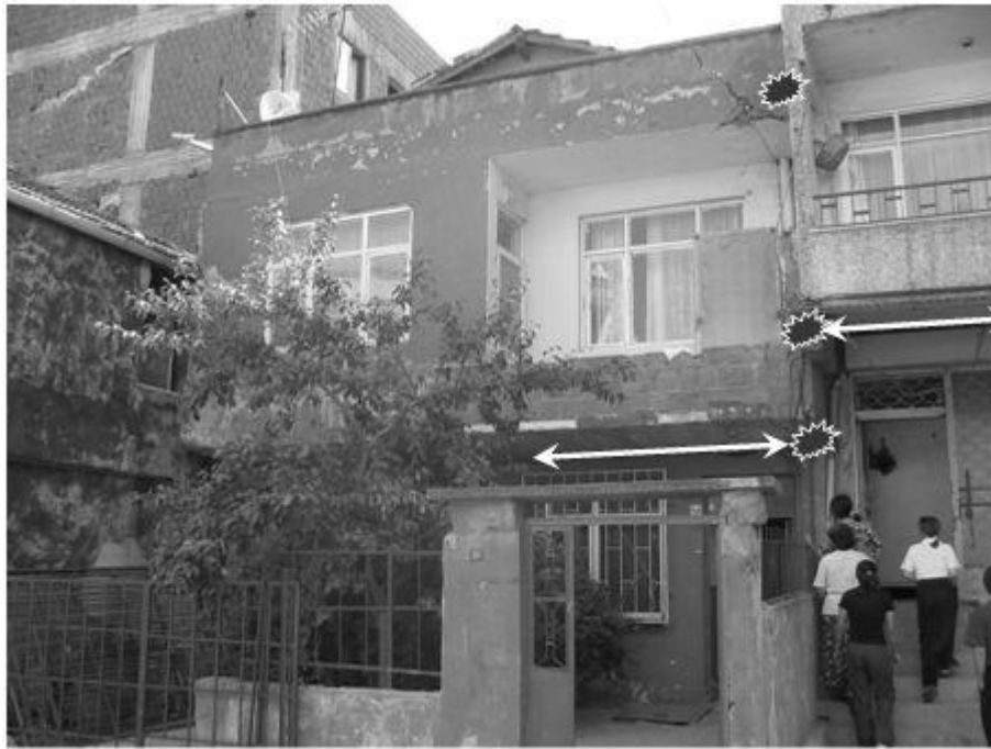
Figure 5. 5. An example masonry building aggregate from Fatih database for which the floor levels of adjacent buildings have different elevations
