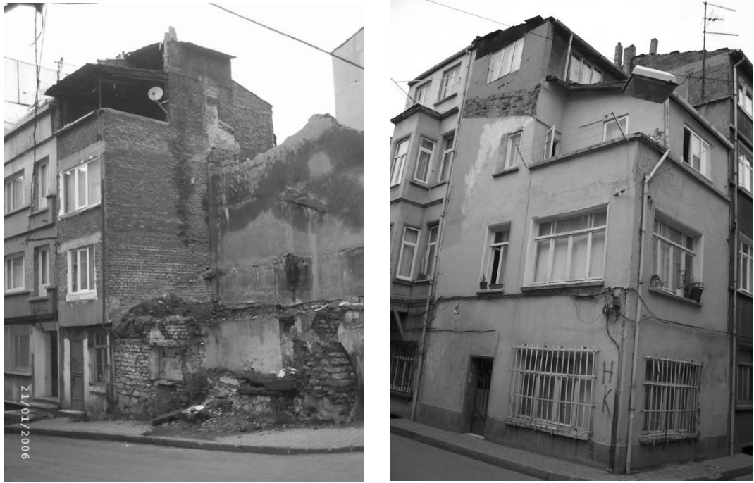
Figure 2. 6. Examples of masonry buildings which do not obey the code regulations in terms of number of stories in Fatih, Istanbul.
