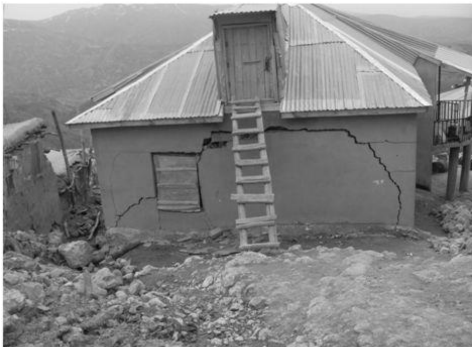
Figure 4. 21. Damaged brick masonry buildings in Okçular village with typical in-plane shear cracks (photos taken by METU-EERC team).
