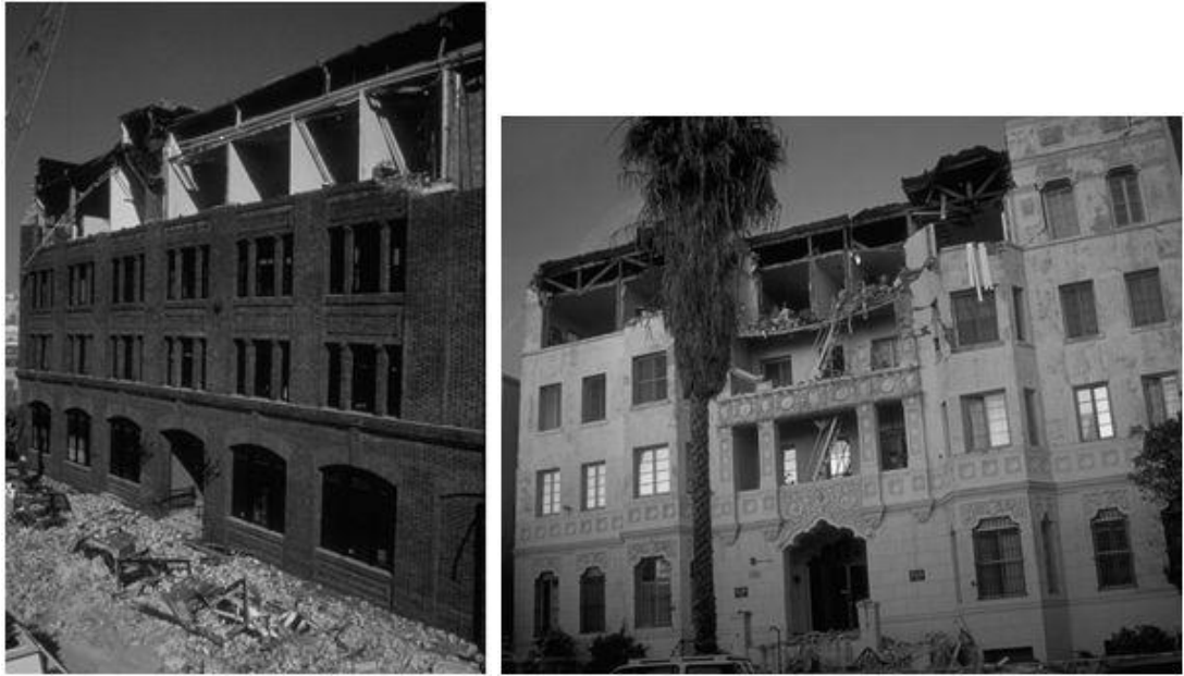
Figure 4. 3. Typical examples for out-of-plane failure of unreinforced masonry walls in the uppermost stories of damaged buildings during a) Loma Prieta earthquake (1989), b) Northridge California earthquake (1994).
