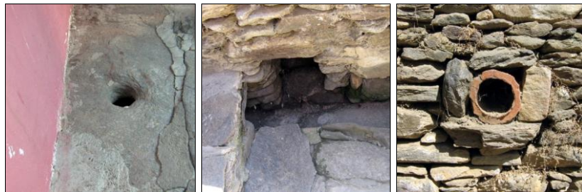
Figure 148, Water drainage system on higher part of taşlık (left), main part of taşlık (middle), exterior masonry wall of taşlık (right) (Gaziumurbey (Demirbaba) Quarter Demirbaba Street No: 35)
