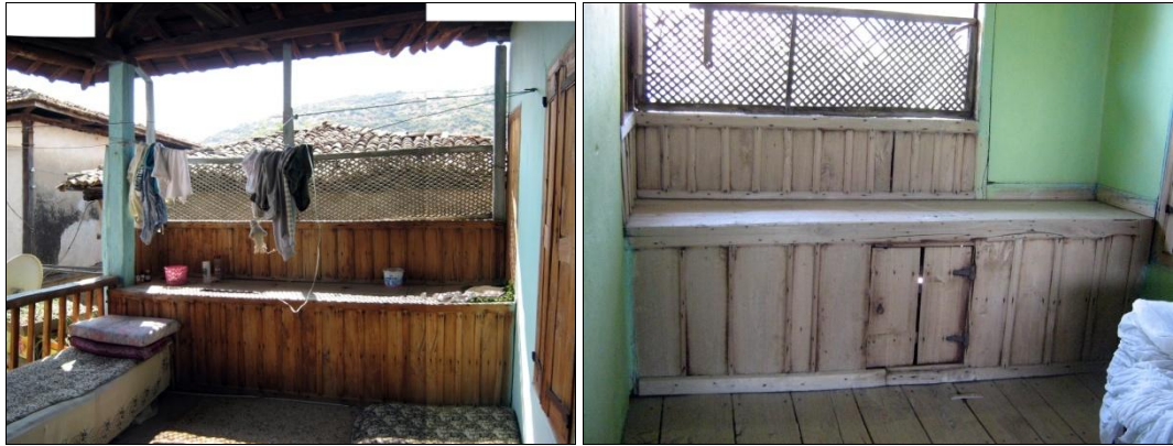
Figure 136, Seki Type 2 – Use of lids on the upper surface (left) (Camikeir Quarter İmam Birgivi Street No:36), Use of lids on the front surface (right) (Camikeir Quarter İmam Birgivi Street No:6)
