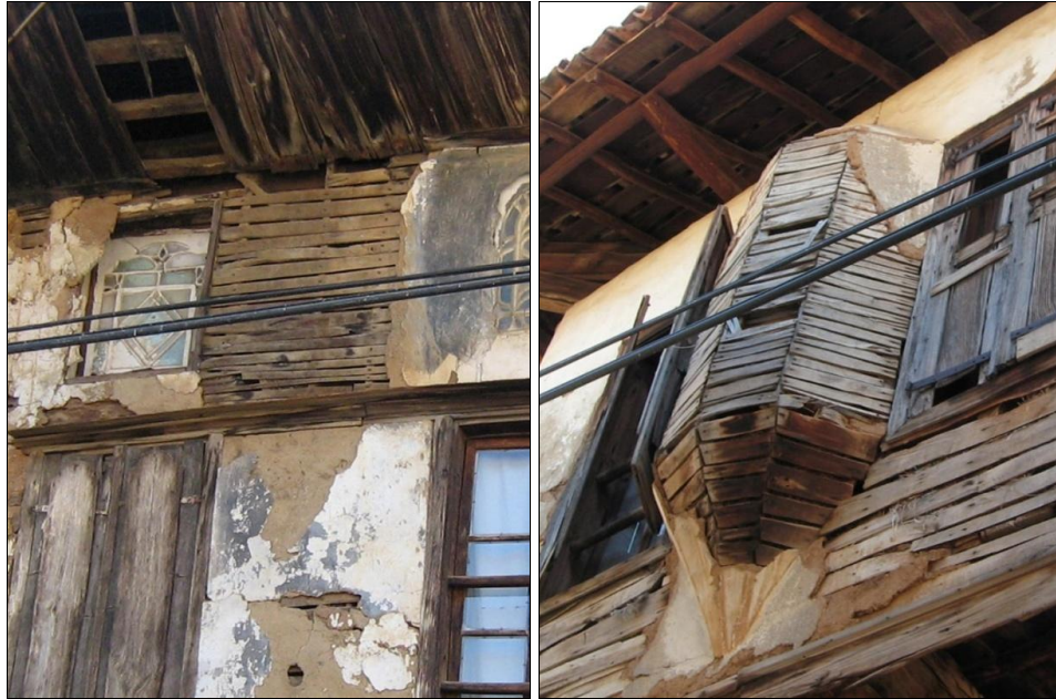
Figure 74, Timber framed wall finishing Type B - Timber lath below the render (Camikebir Quarter Meydanbaşı Street Lot No: 677, Camikebir Quarter İmam Birgivi Street No:36)
