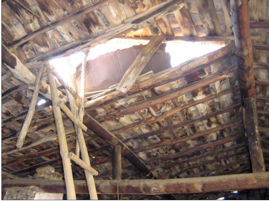
Figure 93, Roof window Detail 1 (Camikebir Quarter Meydanbaşı Street No:13)
