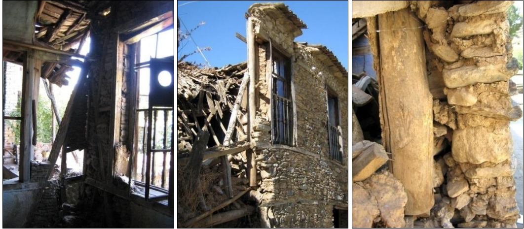
Figure 68, Timber framed wall Type 3 (Camikebir Quarter Okul Street No:2)
