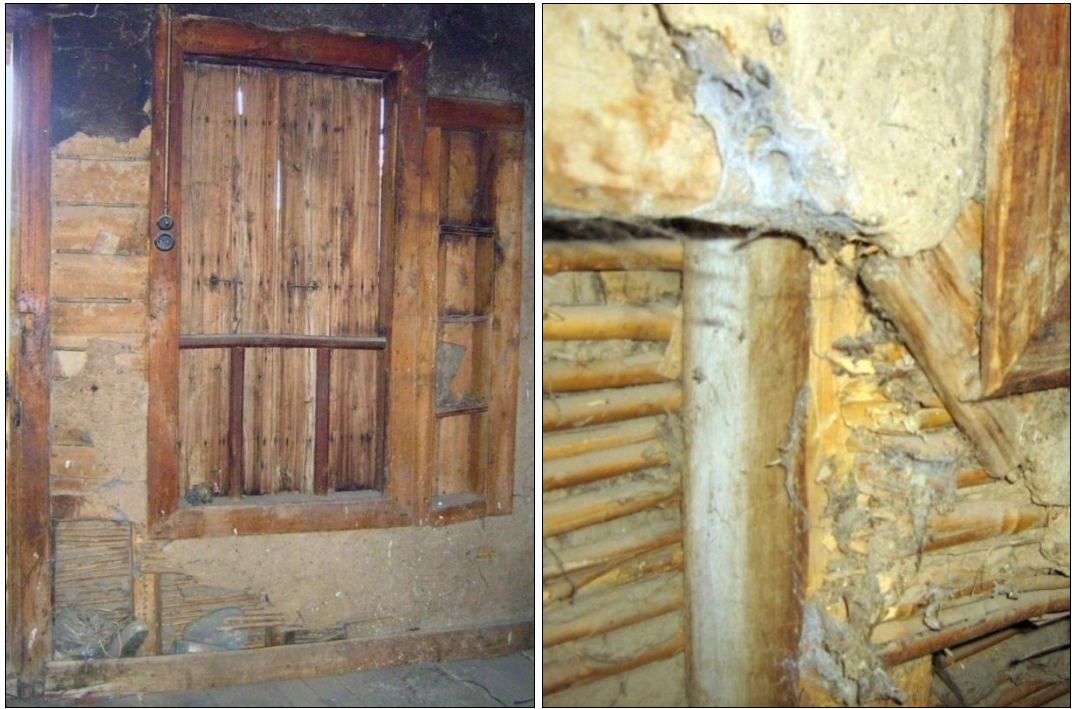
Figure 76, Timber framed wall finishing Type D (Kurtgazi Quarter 3 Eylül Street No:6)
