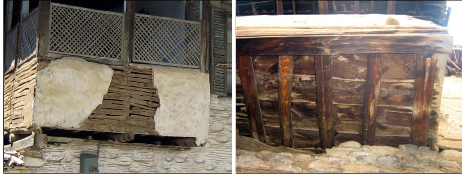
Figure 114, Simple console projection – projection made with girders (left) (Kurtgazi Quarter Şehit Gürol Madan Street No: 78), projections made with floor girders (right) (Camikebir Quarter Karanfil Street No:23)
