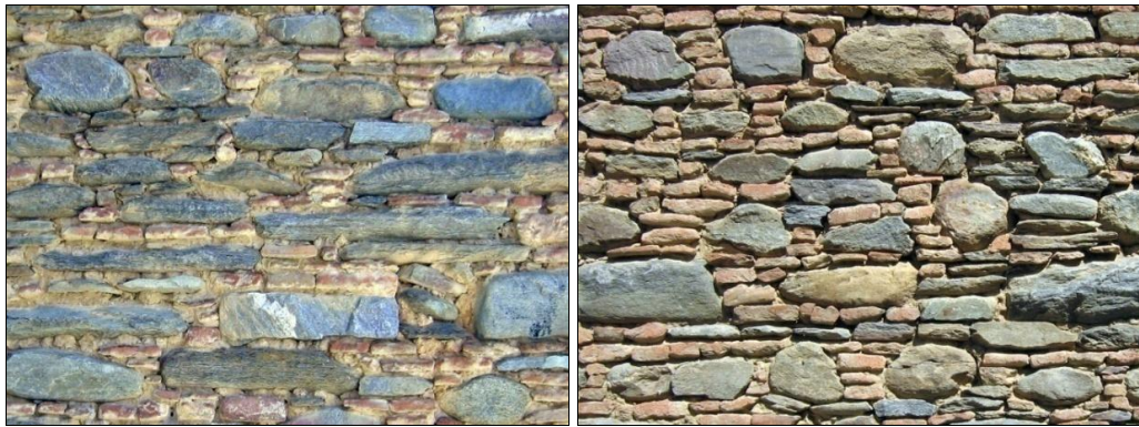
Figure 52, Examples to semi alternating walls
