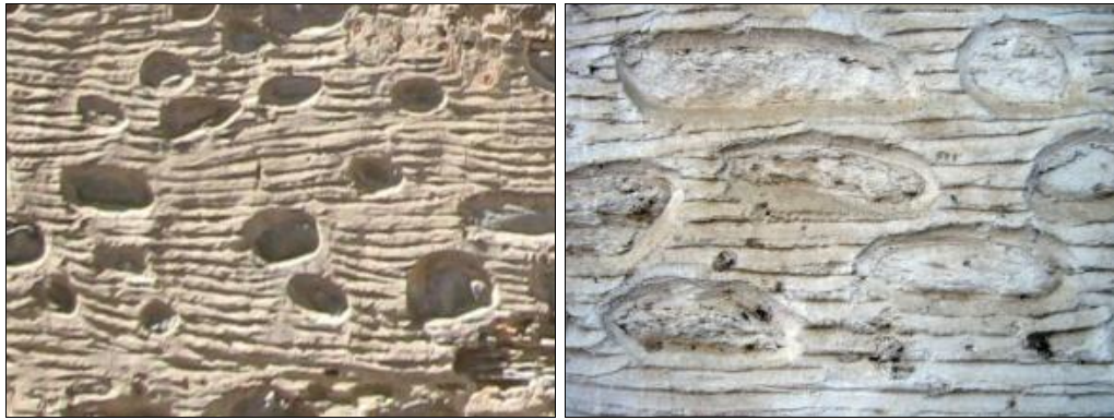
Figure 54, Plastering technique seeming like pointing mortar joints
