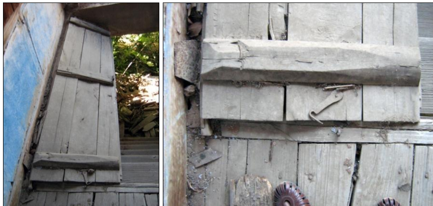
Figure 123, Leaf and hook lock detail used to close the stairs openings (Camikebir Quarter Okul Street No:2)
