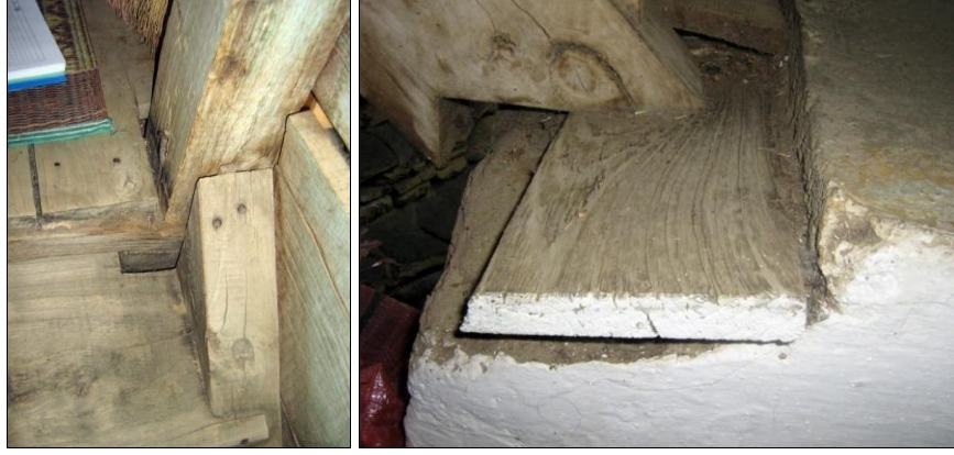
Figure 121, Upper and lower connections of the string belonging to the stairs used between the ground floor and first floor (Cumhuriyet Quarter Umurbey Street No:23)
