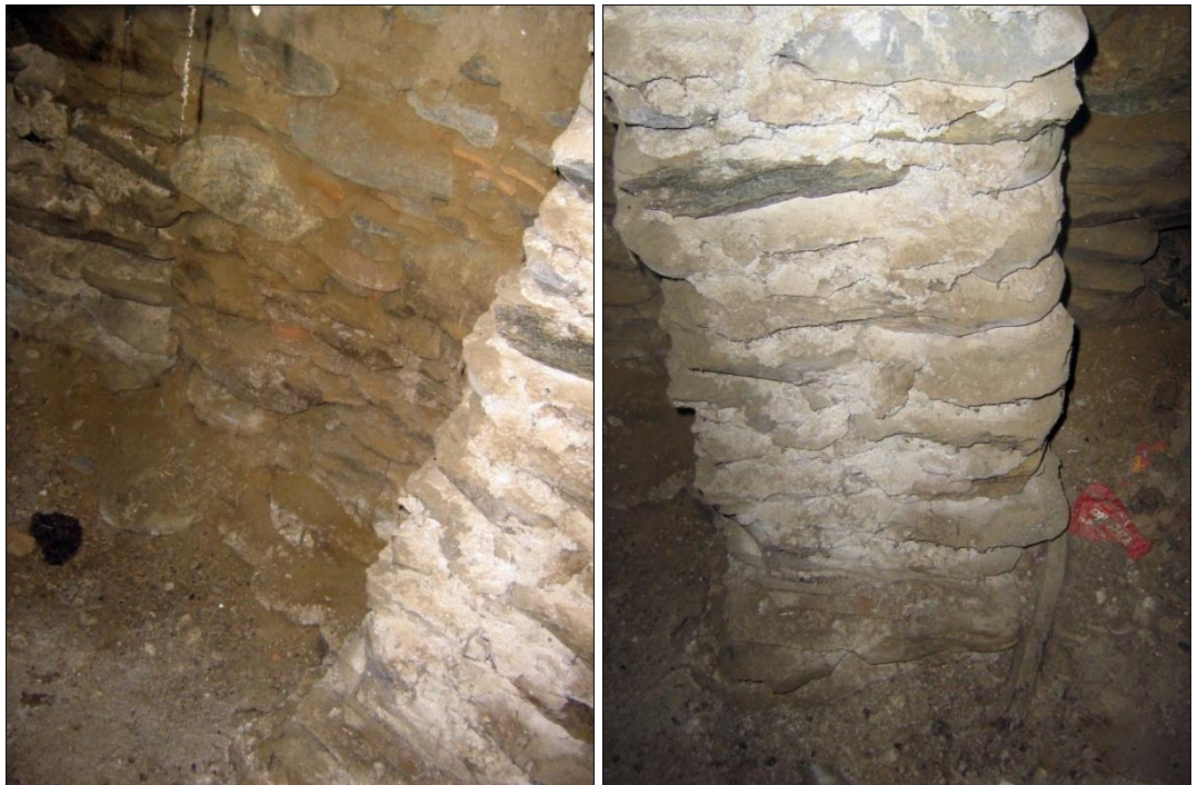
Figure 44, Composite foundation (Camikebir Quarter Camiönü Street No:20)
