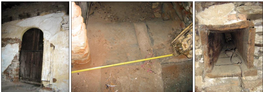
Figure 152, Door openings Type 3 (Camikebir Quarter 3. Beyzade Street No:15) – taşlık façade (left), stone threshold (middle), timber mortise lock housing (right)
