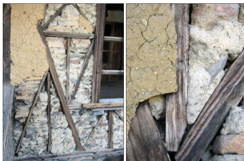
Figure 66, Timber framed wall Type 2 (Camikebir Quarter 3. Beyzade Street No:15)
