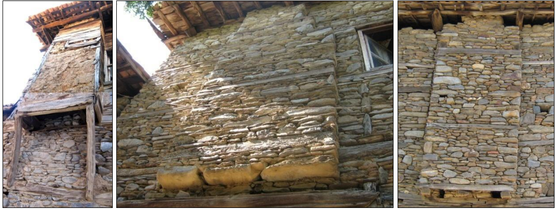
Figure 125, Fireplace projections – fireplace projection sitting on girders and supported by braces (left), fireplace projection sitting on slates (middle), fireplace projection sitting on girders (right)
