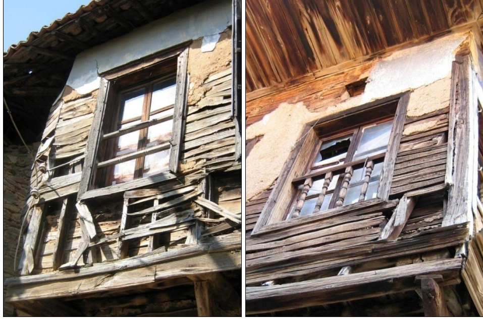
Figure 71, Timber framed wall finishing Type B without infill - Timber plank below the render (Kurtgazi Quarter Ufuk Street No: 4, Camikebir Quarter Meydanbaşı Street No:1)
