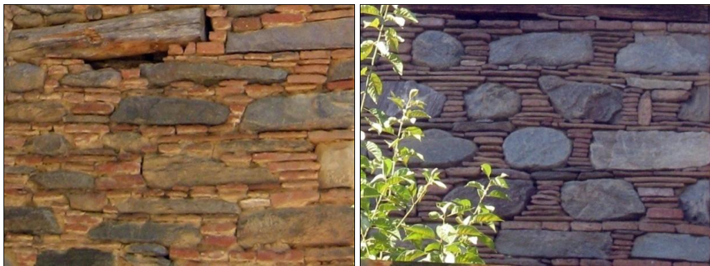
Figure 53, Examples to alternating walls
