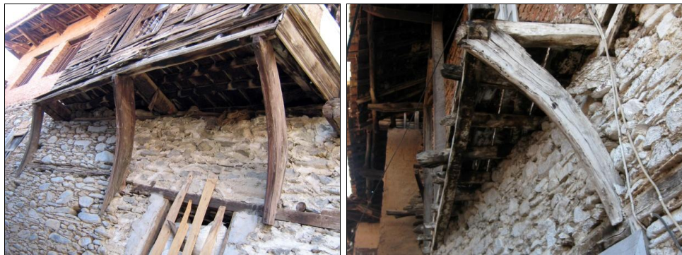
Figure 116, Braced projection – projection with girder, eliböğründe and lower projection sill (left) (Camikebir Quarter Meydanbaşı Street No:1), projection with floor girder, eliböğründe and lower projection sill (right) (Camikebir Quarter Karanfil Street No:12)
