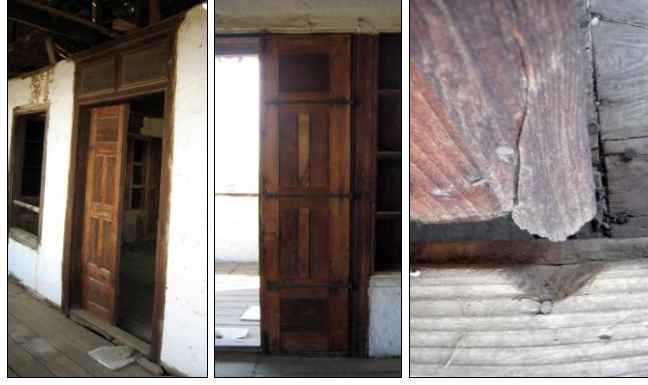
Figure 153, Door openings Type 4 (Camikebir Quarter 3. Beyzade Street No:15) –exterior elevation (left), interior elevation (middle), timber threshold and timber wing connection (right)
