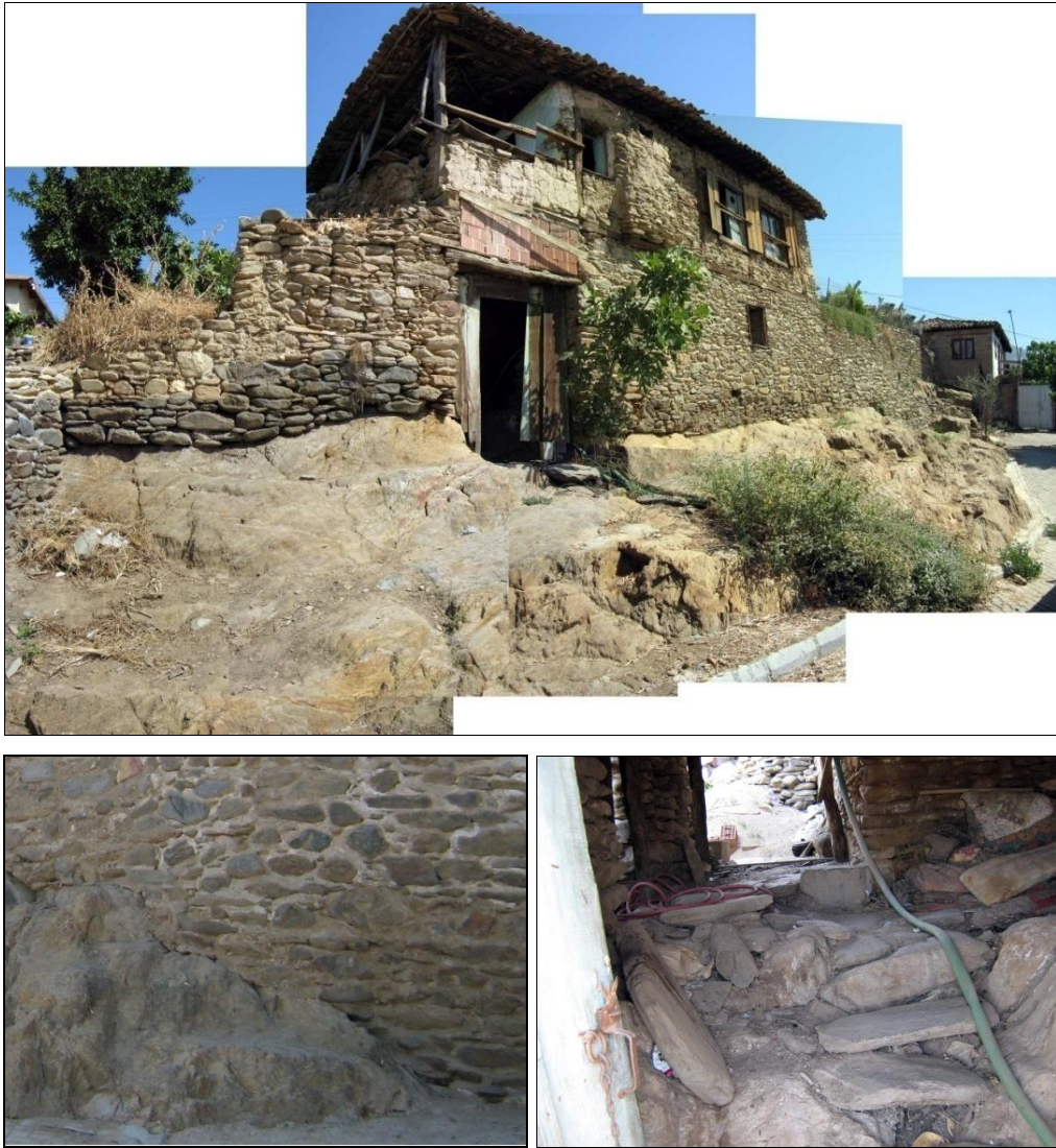
Figure 45, Living rock as a part of the foundation (Kurtgazi Quarter 3 Eylül Street Lot No:1301)
