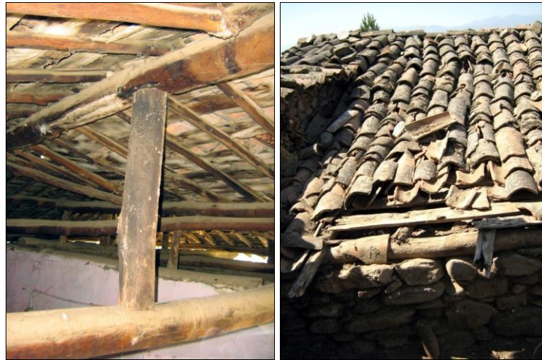
Figure 87, Roof elements –girder, post, purlin, rafter, and roof board relation (left) (Camikebir Quarter Meydanbaşı Street No:13), end purlin, rafter, roof board, and over & under tile relation (right) (Kurtgazi Quarter)
