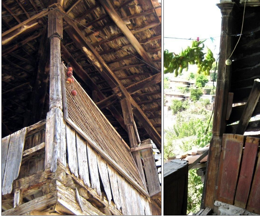
Figure 78, Fine cut timber posts (Camikebir Quarter Meydanbaşı Street No: 1, Kurtgazi Quarter Ufuk Street No: 5)
