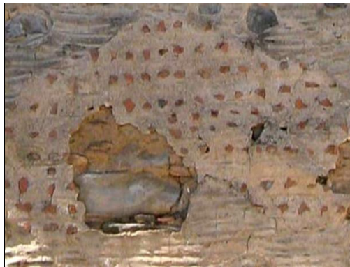
Figure 55, Plastering technique with pieces of brick
