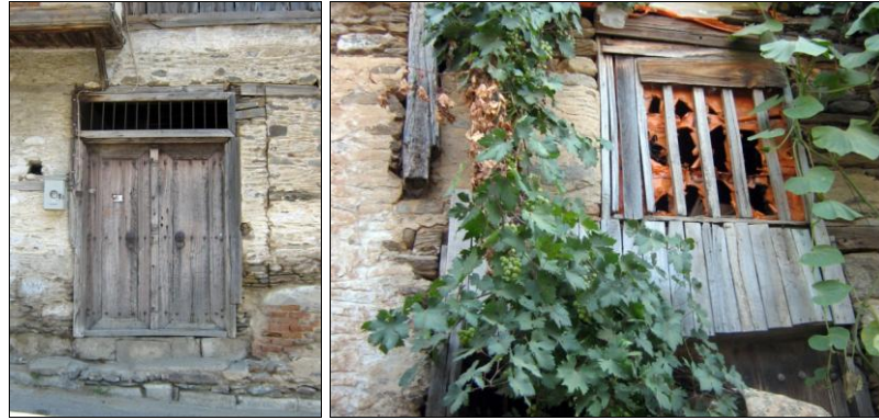
Figure 151, Door openings Type 2 – example of door top window with metal balustrade (left) (Camikebir Quarter İmam Birgivi Street No:6), example of door top window with timber balustrade (right) (Kurtgazi Quarter Ufuk Street No:16)
