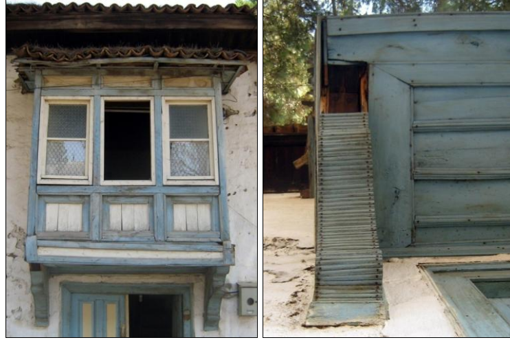
Figure 117, Example to projection covered with profiled planks and timber laths (Cumhuriyet Quarter Umurbey Street No:27)
