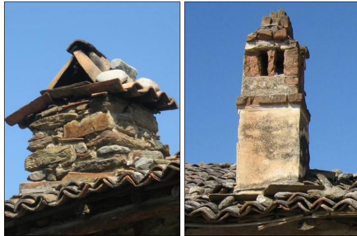
Figure 91, Examples of chimneys – rubble stone masonry chimney caps made of over & under tiles (left), brick masonry chimney (right)
