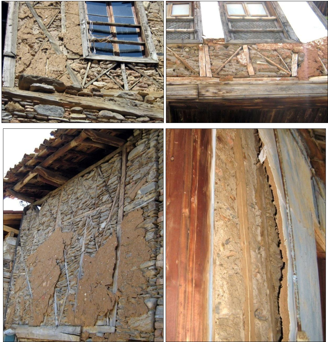
Figure 69, Examples of timber framed wall finishing Type A - Mud plaster
