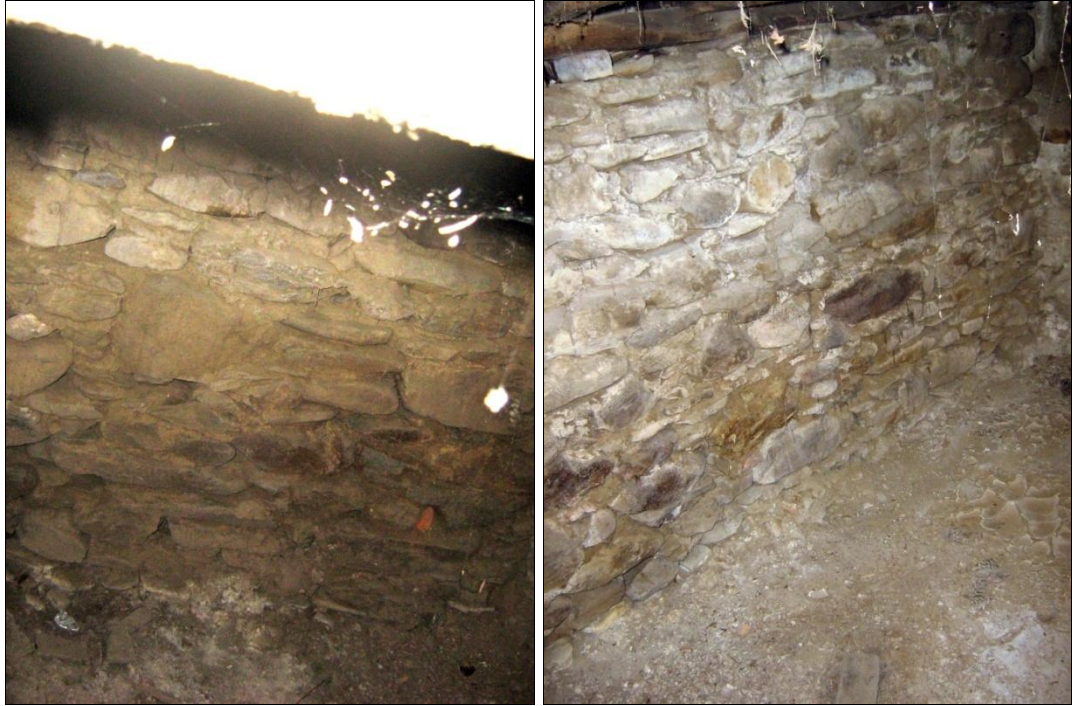
Figure 43, Continuous foundation (Camikebir Quarter Okul Street No:3)
