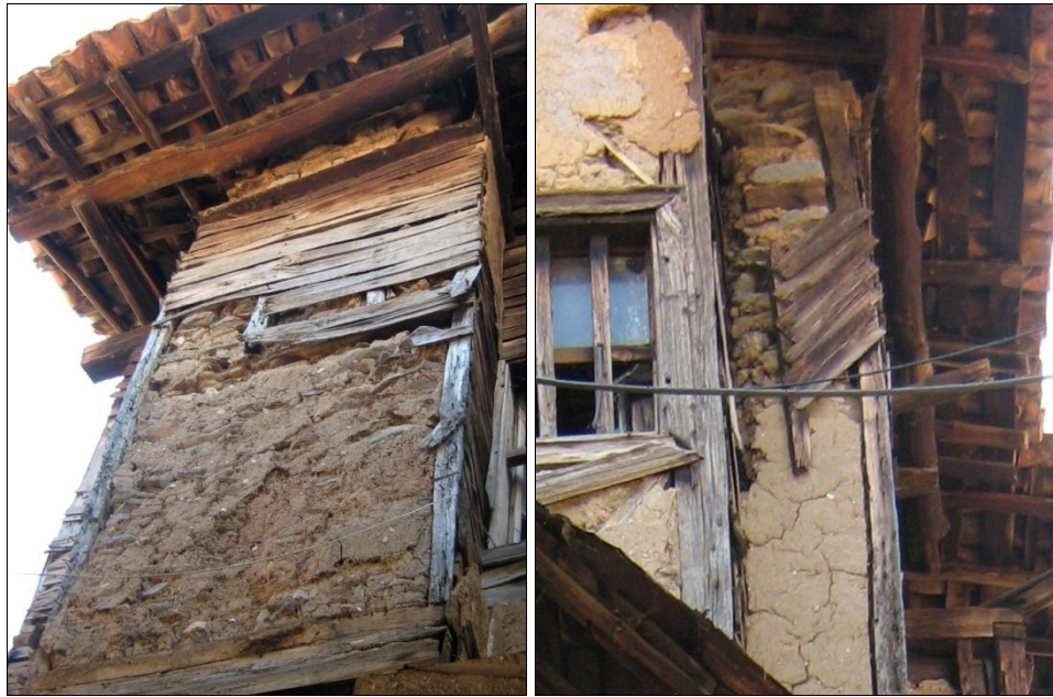
Figure 72, Timber framed wall finishing Type B with infill - Timber plank below the render (Camikebir Quarter 3. Beyzade Street No:31)
