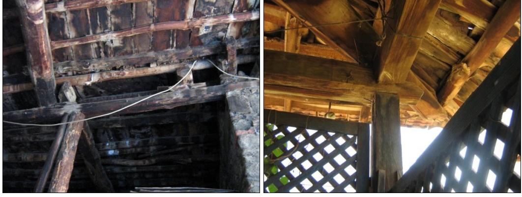
Figure 80, Examples of timber post Detail 1 – Plain connection- taşlık post (left) (Gaziumurbey (Demirbaba) Quarter Demirbaba Street No: 35), sofa post (right) (Kurtgazi Quarter Hıdırbey Street No: 14)
