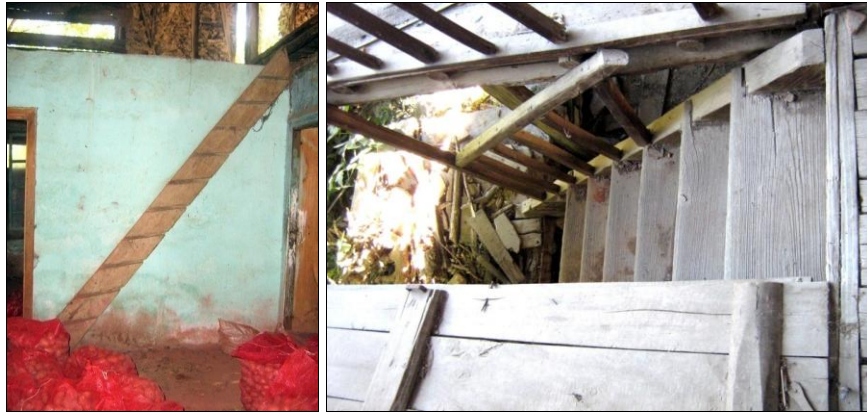
Figure 122, Tread slots where string and steps are placed (left) (Camikebir Quarter Okul Street No:3), stringer and treads (right) (Camikebir Quarter Okul Street No:2)
