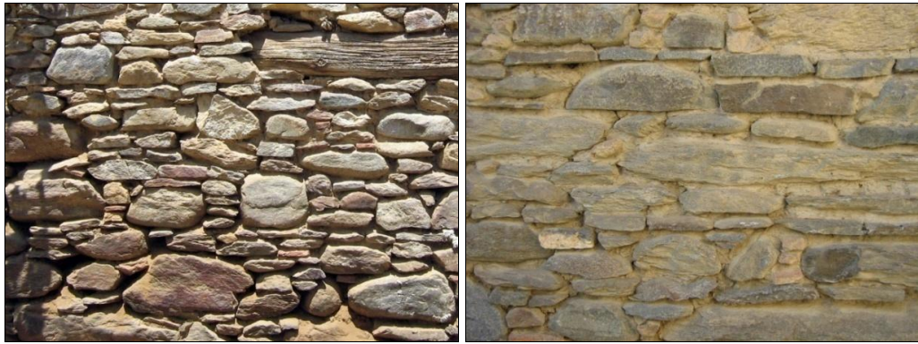
Figure 51, Examples to coursed rubble stone masonry walls
