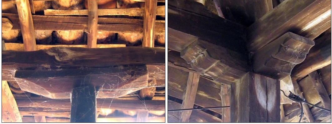
Figure 81, Examples of timber post Details 2 - Post with bolster on top – Posts located in sofa (left, Kurtgazi Quarter Ufuk Street No: 16), (right, Camikebir Quarter Meydanbaşı Street No: 1)
