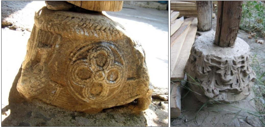
Figure 79, Use of spolia as plinths of timber posts (Camikebir Quarter 1. Beyzade Street No:10, sağda Camikebir Quarter 3. Beyzade Street No:15)
