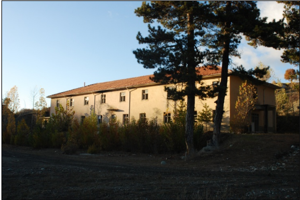
Figure 10 Abandoned administration building
