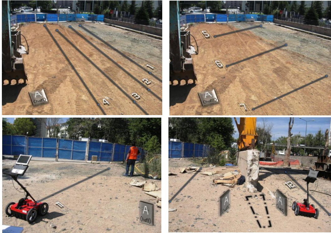
Figure 3.19. Region A, Line 1, Line 2, Line 3 and Line 4 profiles (profile number 1, 2, 3, 4, 5, 6, 7, 8, 9, 10, 11, 12).
