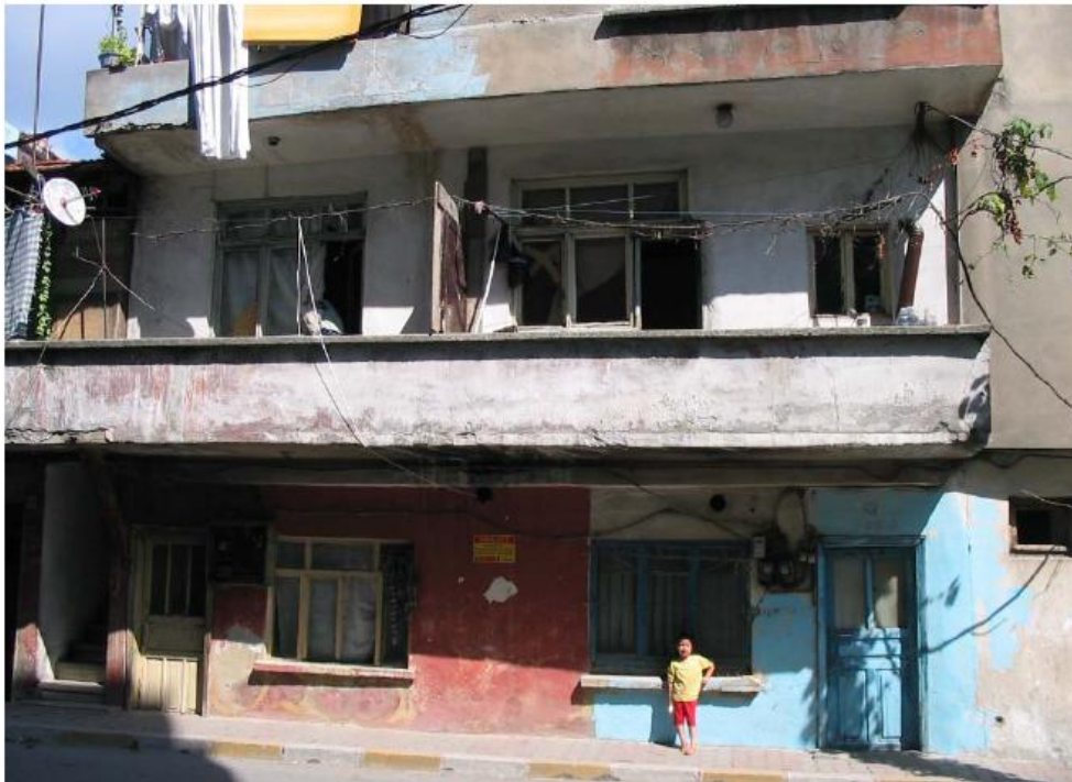
Figure 5.37. Picture of the masonry building used as a case study
