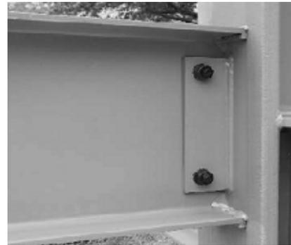
**Figure 4.7** Single plate connections.
