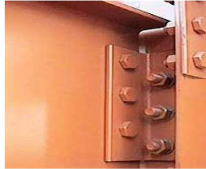
**Figure 4.6** Single web-angle connections.
