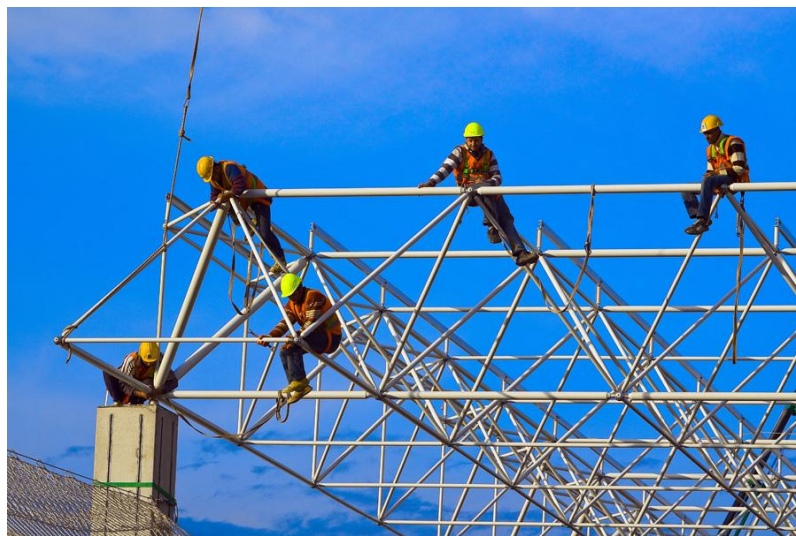
Figure – 1: Double-layer grids under construction
