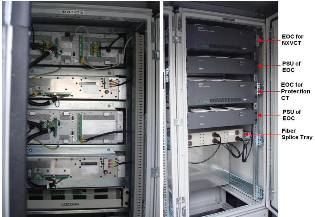
Figure 2.26: The Electronic System - Back and Front View of the Cabinet
