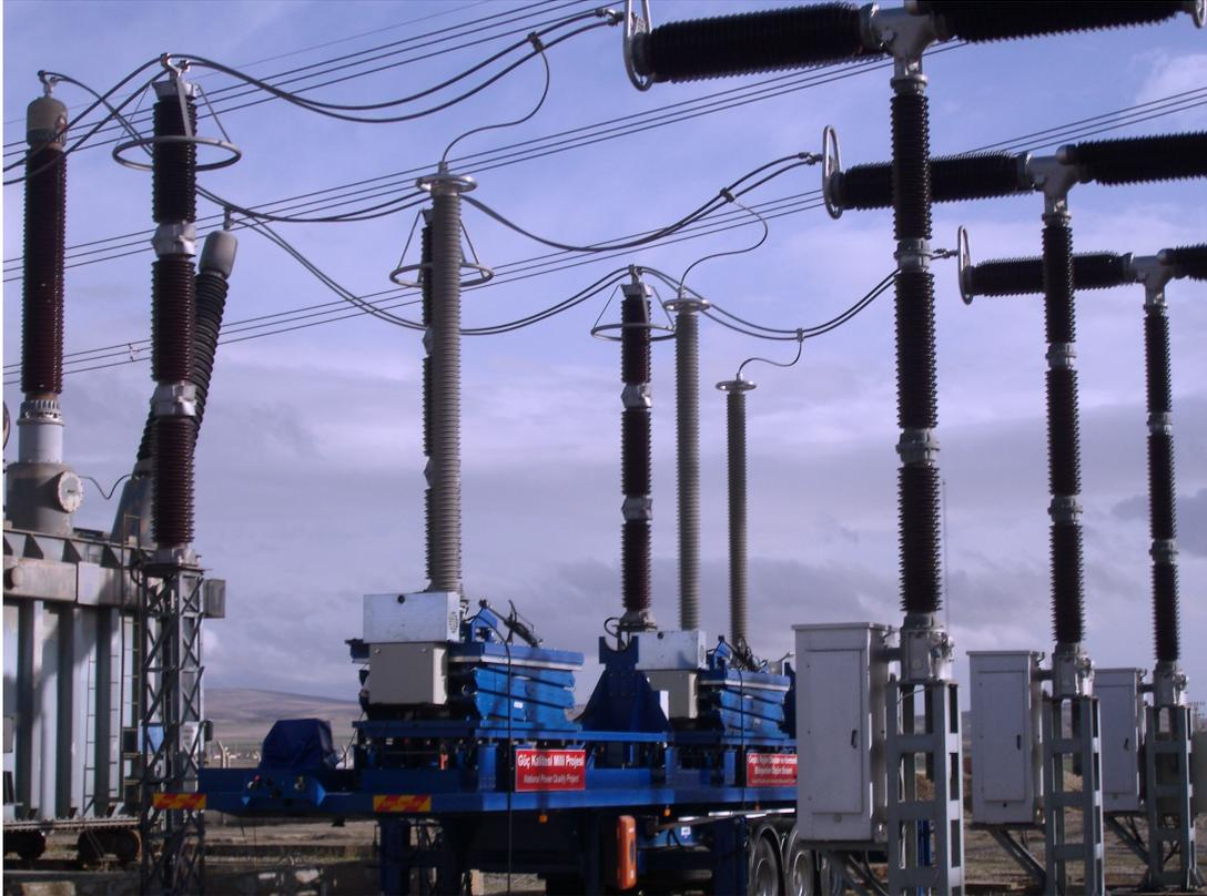
Figure 2.13: 420kV RCVT in the substation of Temelli in Ankara
