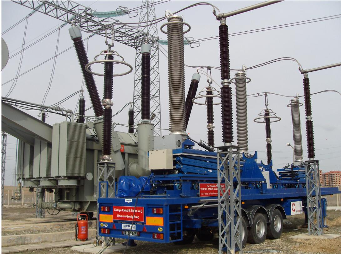
Figure 2.22: 420 kV NXVCT at substation of Temelli in Ankara
