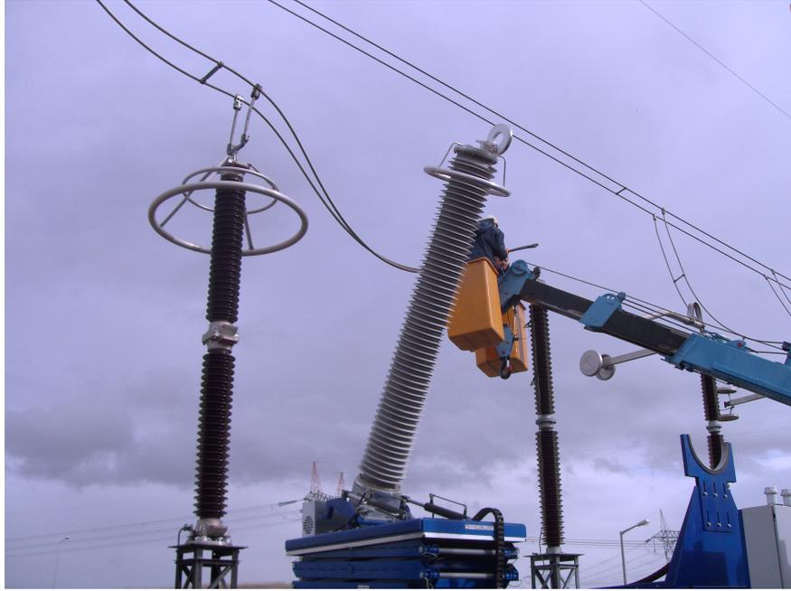
Figure 3.2: 420 kV NXVCT column while tilting up for connection
