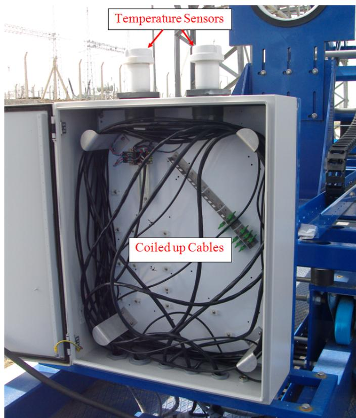
Figure 3.7: Temperature Sensors and Coiled up Cables
