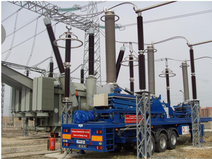
Figure 3.3: 420 kV NXVCT column is tilted up
