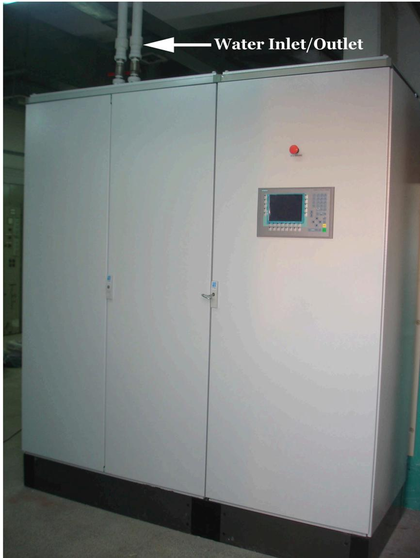
Figure 5.16: IGBT and control panels after installation
