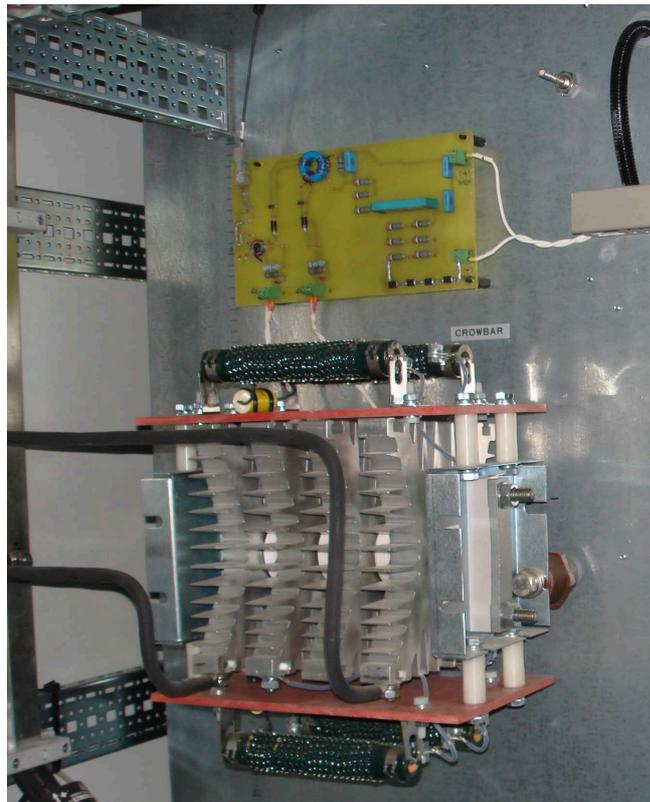
Figure 4.39: A sample picture of the implemented crowbar
