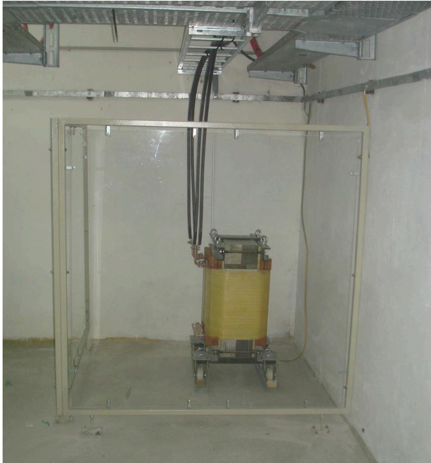
Figure 5.19: Sample view of dc-link reactor after installation
