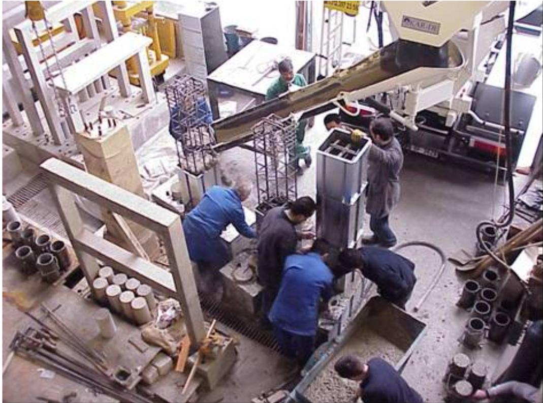
Figure 3.6 Concrete placing for a Type-2 column with ready-mixed concrete
