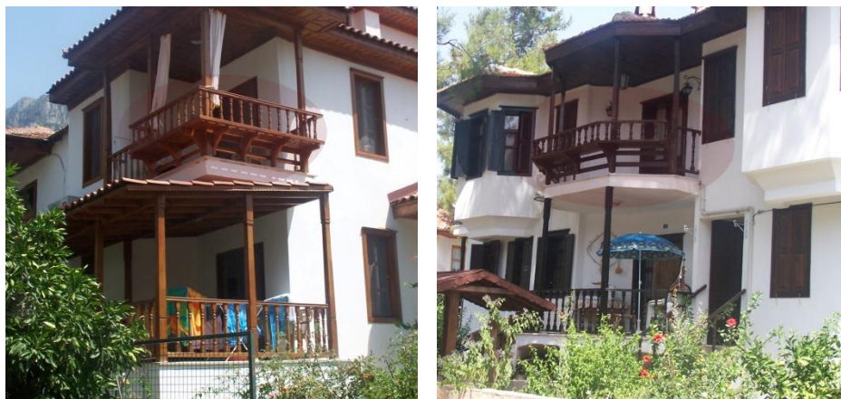
FIGURE 4.39. The balconies with timber railings, which are in the form of sitting desk are very common in houses. Source: Photographs taken by the author (during the visit in Akyaka, July 2008)
