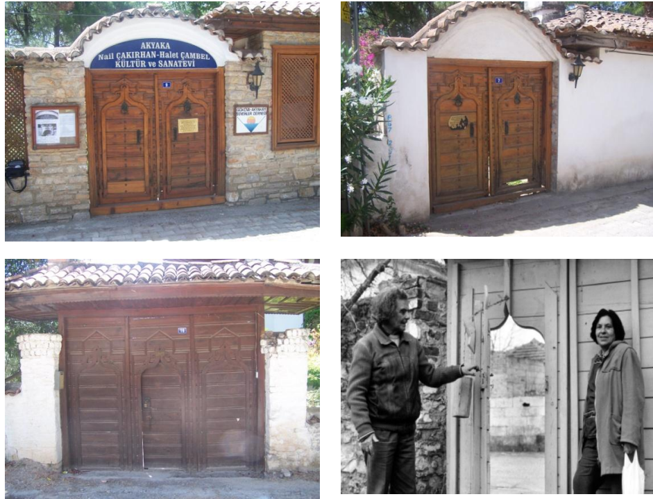
FIGURE 4.37. “Kuzulu Kapı” Entrances by Çakırhan. It is a traditional entrance door which has a smaller wing in it that makes the visitor to bend which symbolizes respectfulness to the house. Source: Photographs taken by the author, right corner below, Aga Khan Records (during the visit in Akyaka, July 2008)
