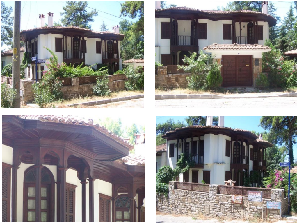
FIGURE 4.27. Büke Sisters Twin House, 1992. Source: Photographs taken by the author (during the visit in Akyaka, July 2008)
