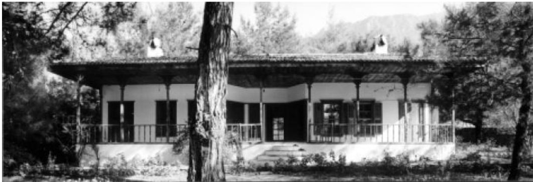
FIGURE 4.2. Çakırhan House South View. Source: Arch Net Web Site, Aga Khan Record Files, Photographs submitted by the architect to document the project. Retrieved December 14, 2010 from ( http://archnet.org/library/files/one-file.jsp?file_id=334 )
