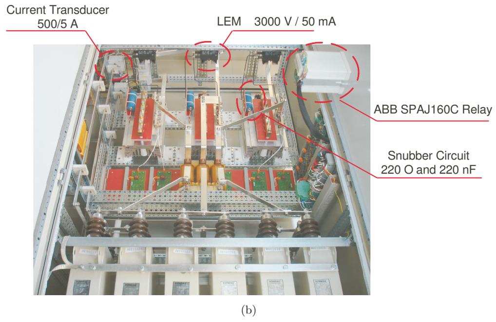
Figure 4.41: Picture of practical cabinet design of TSC. (a) View 1, (b) View 2.
