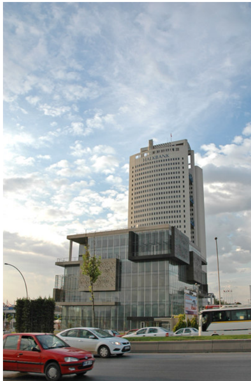
Figure 4.23 DMC Building. Photographed by the author.
